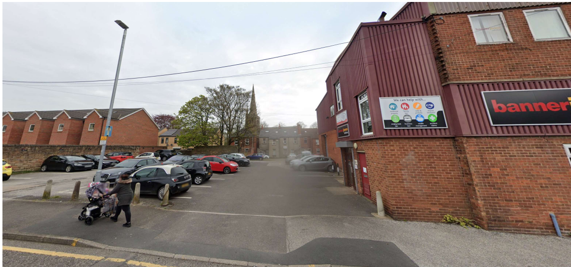
View of Rear of Building from Union Street
