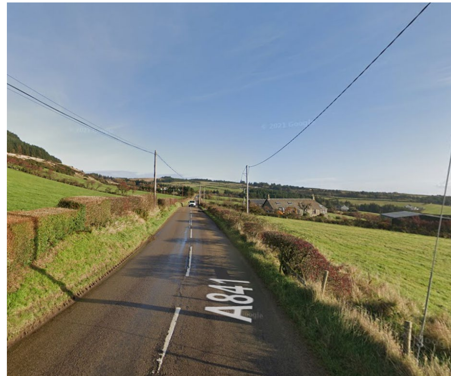
Figure 4. Looking east on A841 from existing site entrance.
