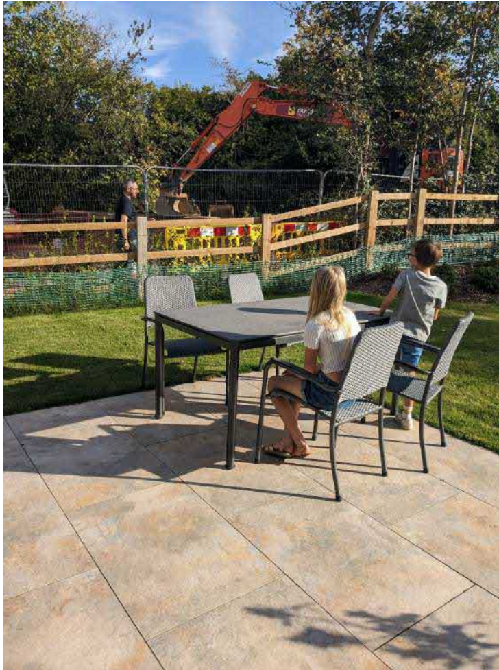
Photo 2: Taken from the rear garden patio of the property. Pedestrian passerby visible on the footpath immediately in front of the garden. Extensive roadworks taking place on New Road demonstrate the proximity to the road. No zoom.
