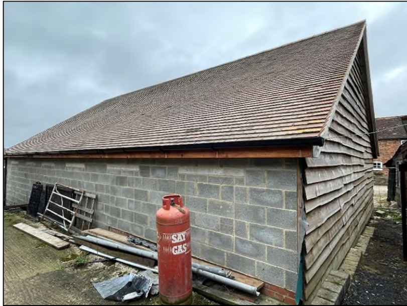
Plate 1: typical view the Barn at Harpers Farm. Photograph looking east.
