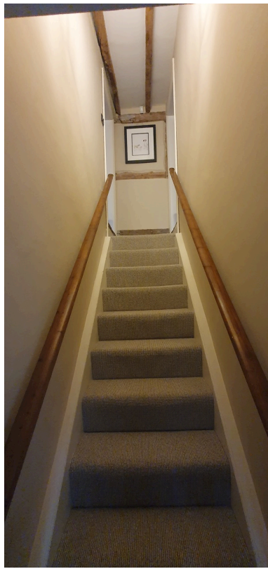
Stairs in both directions showing large painted timber cover strips on the strings to both sides
