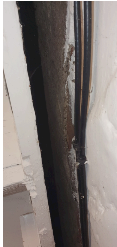
Underside of these stairs showing they are modern poor quality and poorly fitted in the space with large gaps to both sides.
