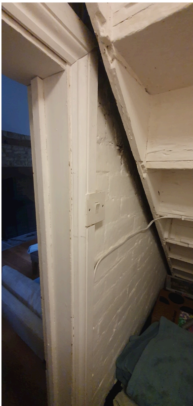
Underside of these stairs showing they are modern poor quality and poorly fitted in the space with large gaps to both sides.
