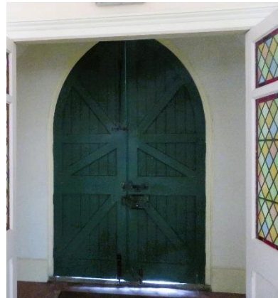
Internal view of inside of front doors
