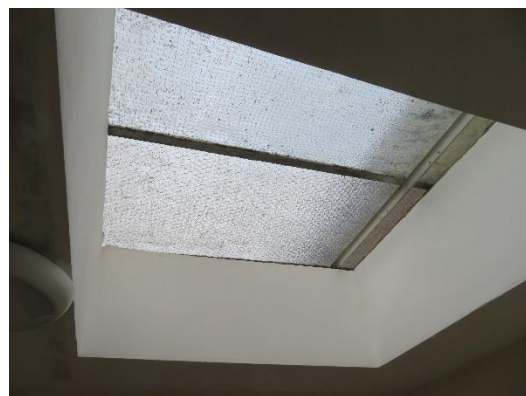
Rooflight with Georgian Wire Glass
