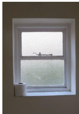
One of two windows in ladies toilet facing north overlooking neighbour's back garden fence/wall
