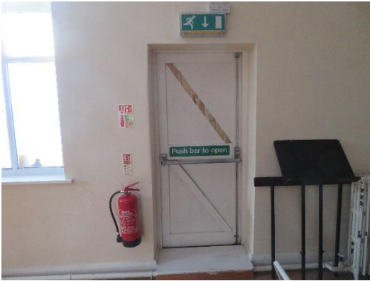
Fire door to rear
