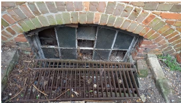
Window from cellar to ground level
