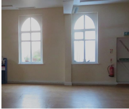
Windows in Hall facing north over neighbour's garden fence
