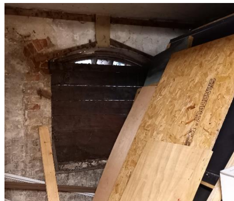
Store room with ground level window
