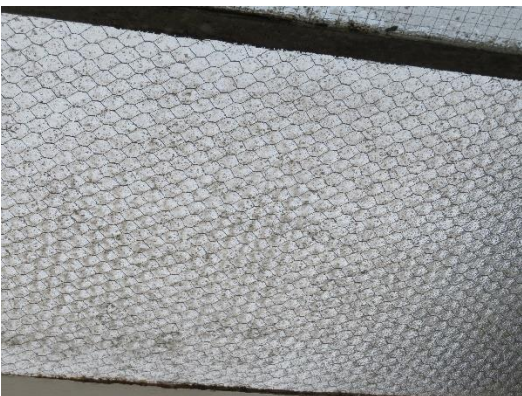
Rooflight with Georgian Wire Glass
