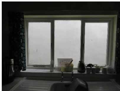
Kitchen window facing east looking at neighbour's wall
