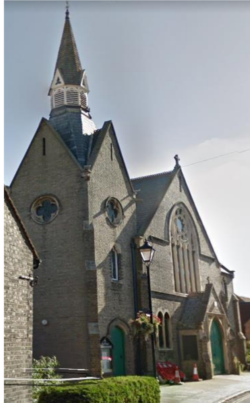
The church from the north west, showing the front entrance with the 1891 front extension.
