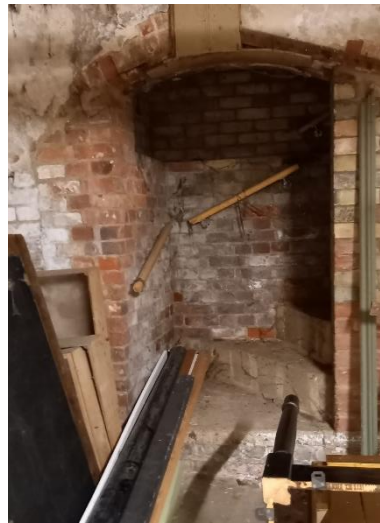
Stairs to South West elevation
