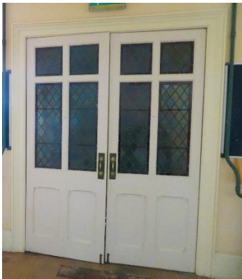
Internal doors to main front doors
