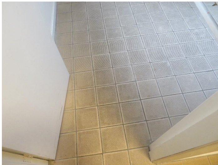
Flooring in both toilets
