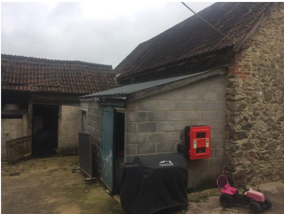
Rear of barn 3 north east
