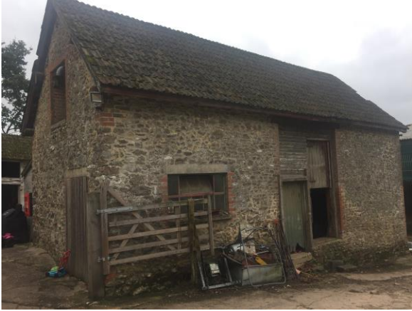
North east elevation (barn 3)
