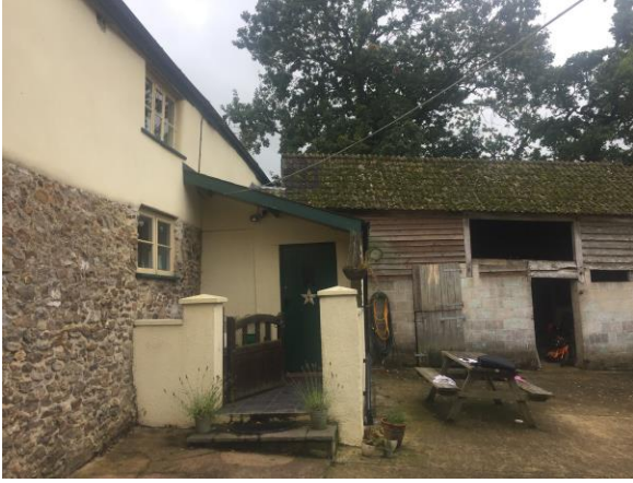
Rear porch with north east elevation of barn 1 in background
