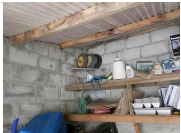
View of the interior of the southern half of the barn, frequently used, bright, showing the intact pointing, and the intact roof.
