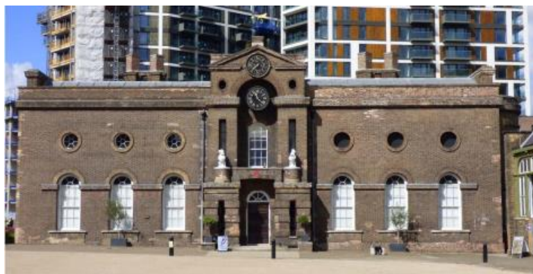
Front façade of Building 40
