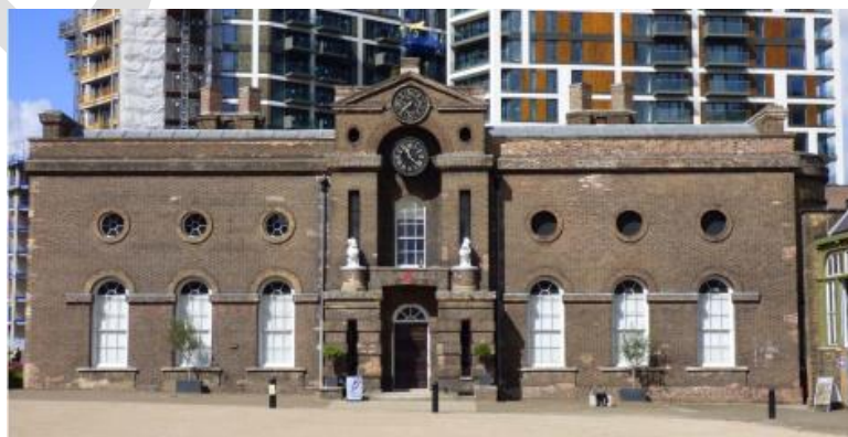
Front façade of Building 40
