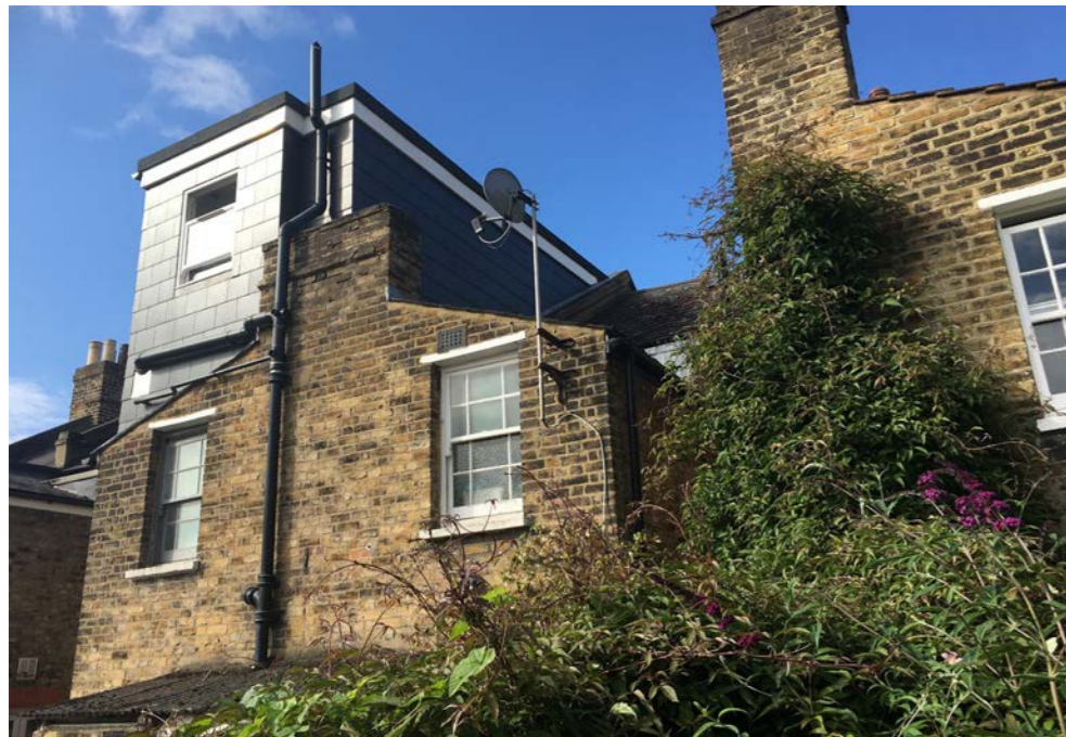
Photograph of extant roof extensions at adjacent dwellings along Rye Road
