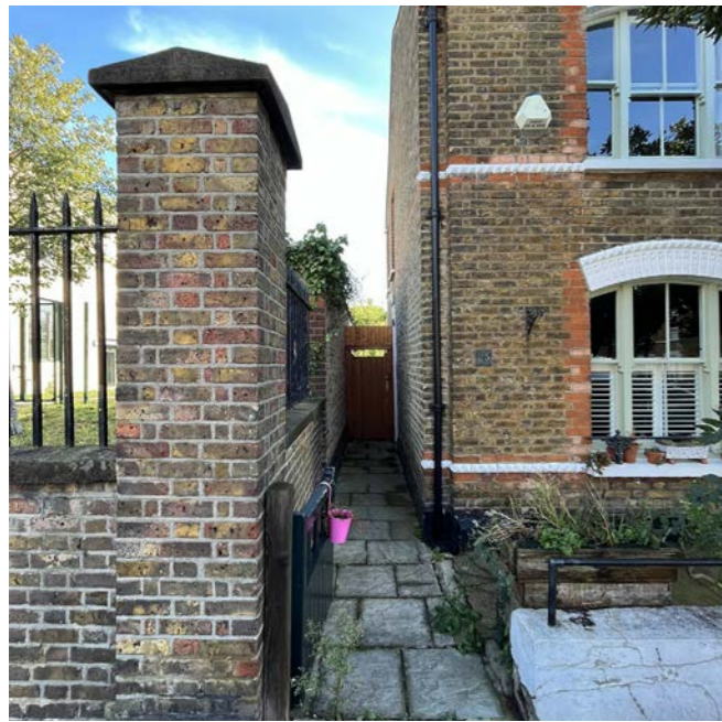
Photograph of existing building
