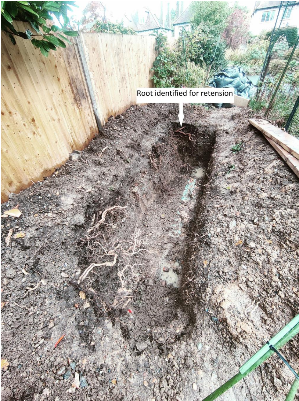
Picture 1 (top left)- showing the trial excavation trench and the root identified for retention at the North end. Very little other rooting activity, with lighter coloured roots not from tree N003.
