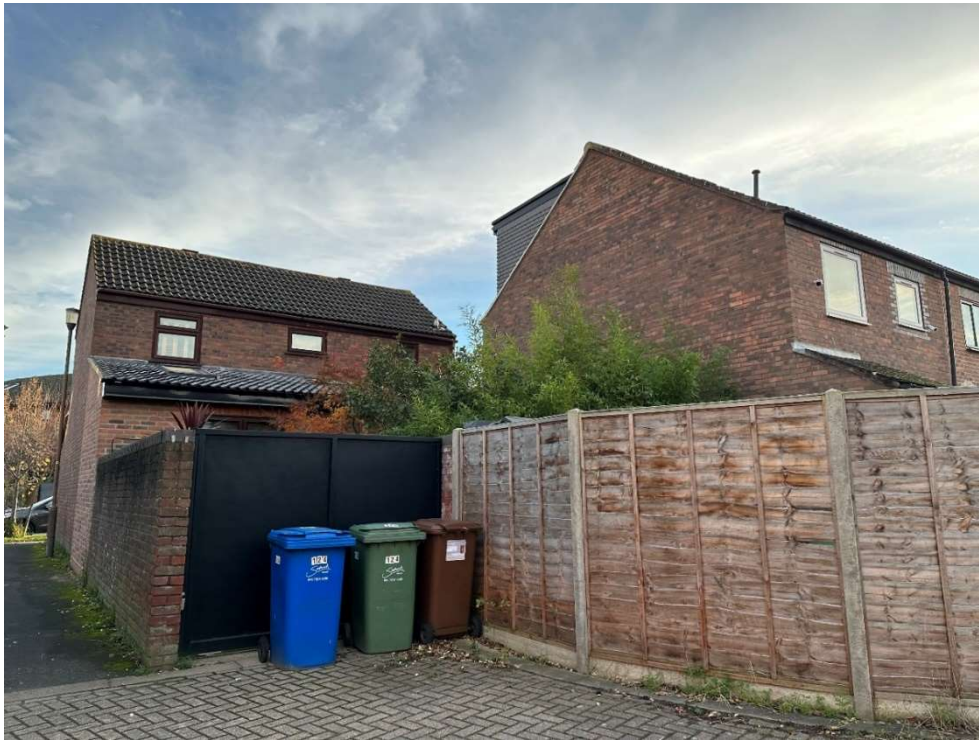
FIGURE 3 - VIEW OF 124 REDRIFF ROAD BOUNDARY WITH NO.14 FRONT GARDEN
