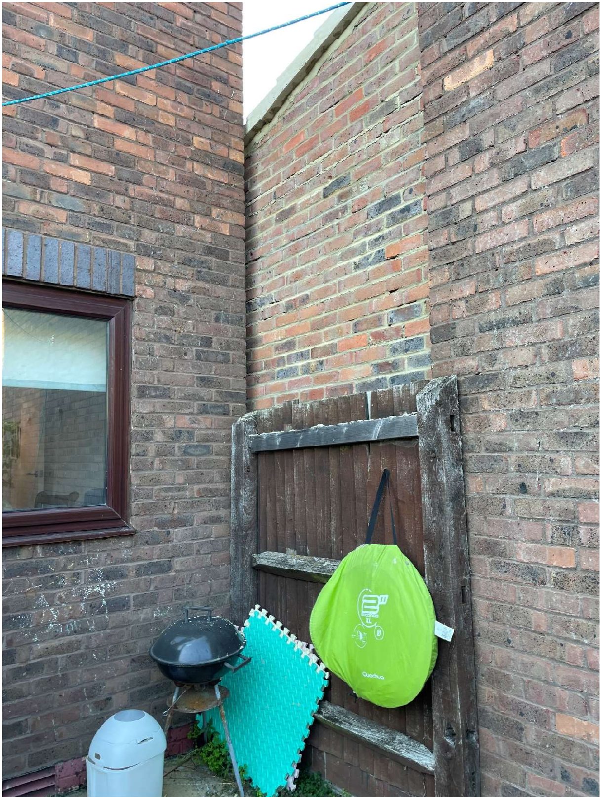
FIGURE 9 - BOUNDARY ABUTTING 124 REDRIFF ROAD NEIGHBOURING WALL AND EXTENSION
