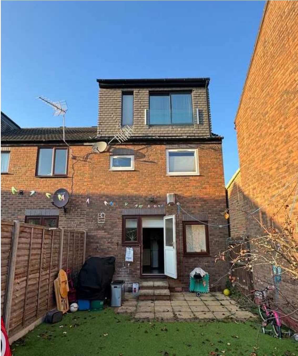
FIGURE 2 - VIEW OF REAR ELEVATION
