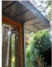
6. Metal cladding to porch/canopy
