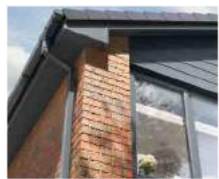
5. Dark grey UPVC rainwater goods & soffits
