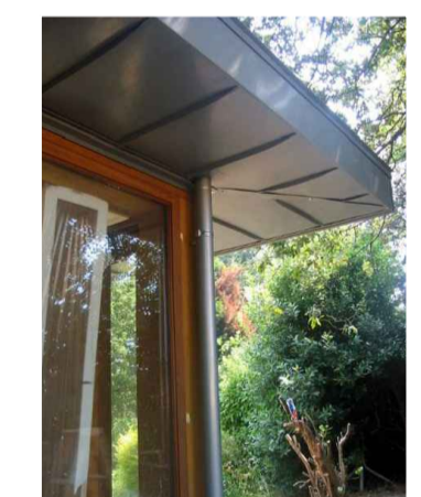
6. Metal cladding to porch/canopy
