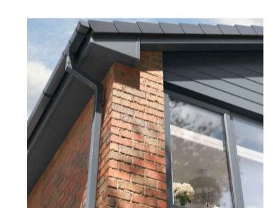
5. Dark grey UPVC rainwater goods & soffits
