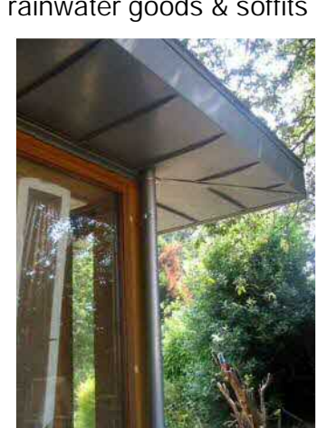
6. Metal cladding to porch/canopy
