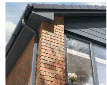
5. Dark grey UPVC rainwater goods & soffits
