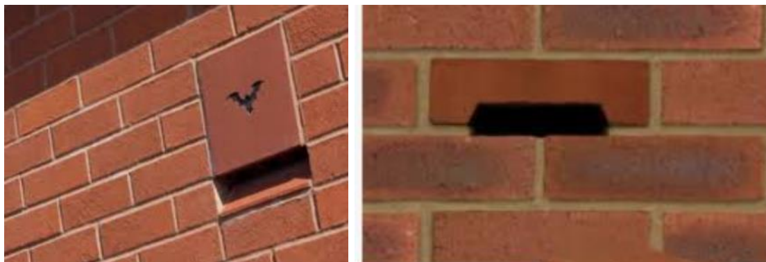
Figure 34. Example of bat bricks in external walls
