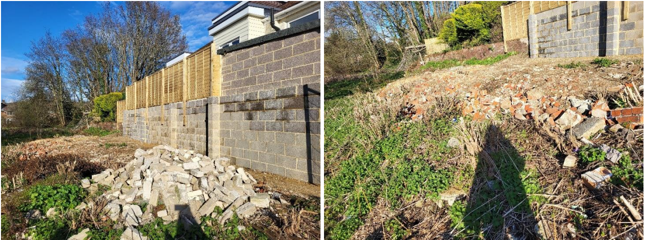
Figure 20. View of the area of bare ground on site (May 2023)
