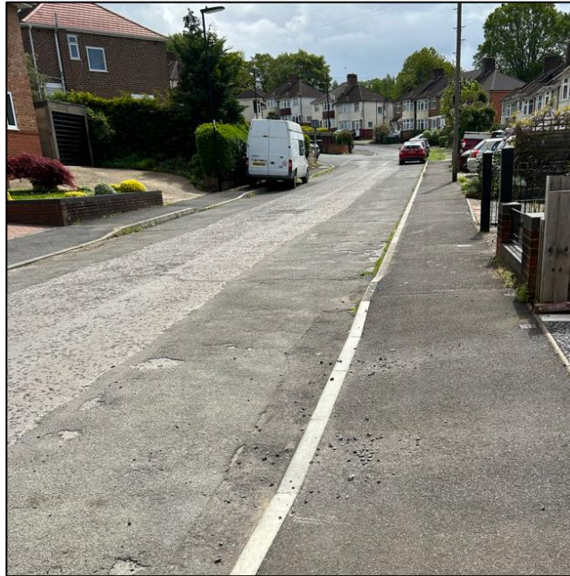
Photograph 2: Existing Footways along Bryanston Road
