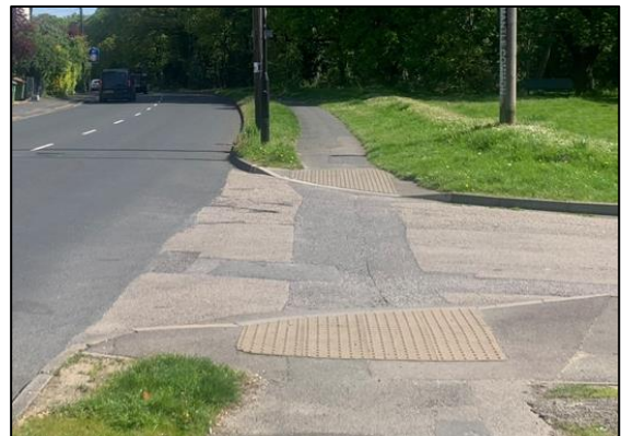
Photograph 4: Dropped kerbs with tactile paving across junctions
