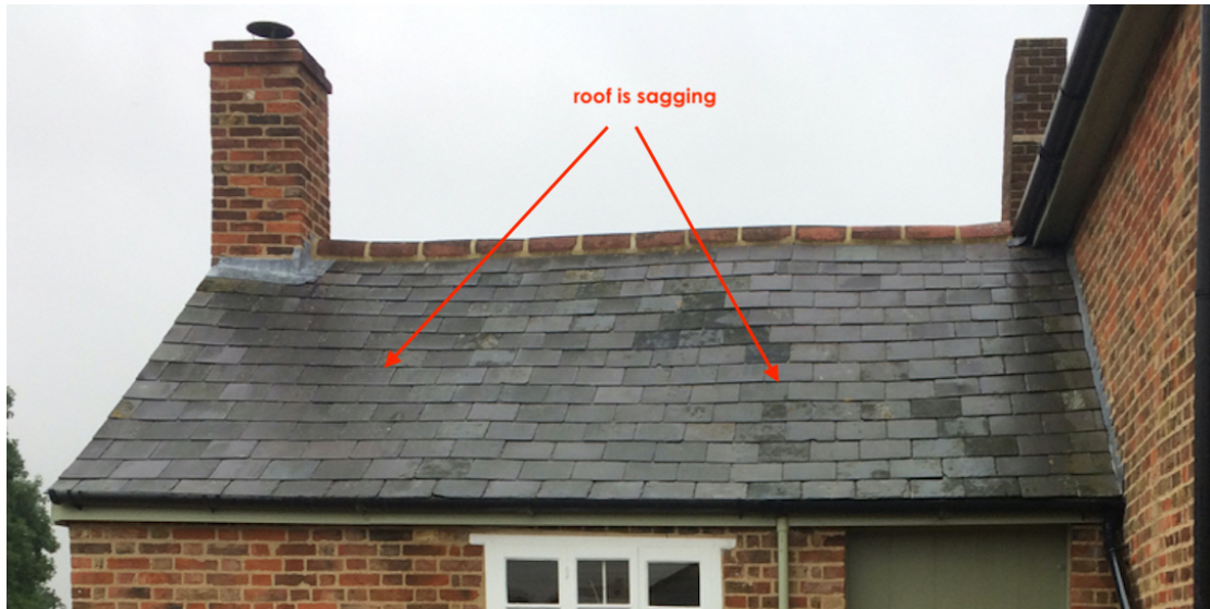
Brewhouse roof Pitch 3
