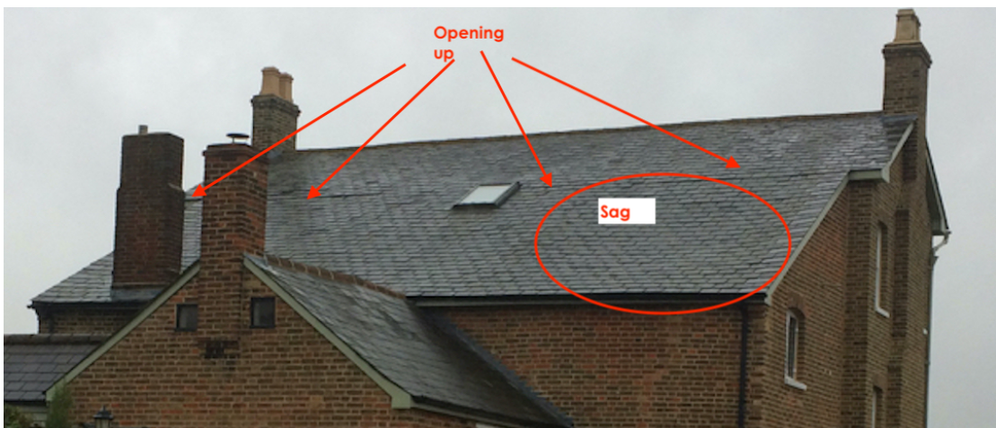
Main roof at rear – Pitch 2
