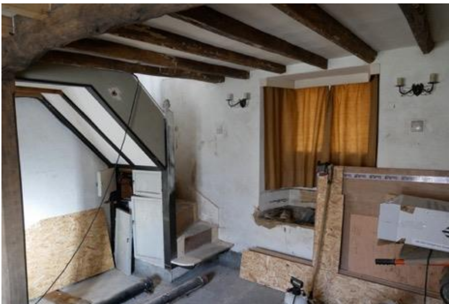
Plate 10: C17 section, ground floor with C20 internal finishes and staircase
