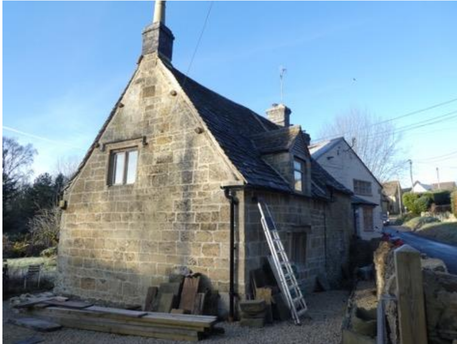
Plate 6: East and north elevations, C17 section to left with lower eaves and C20 dormer
