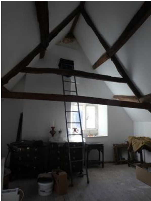
Plate 11: C17 section, first floor looking east with single truss, double purlin construction and a secondary collar at low level
