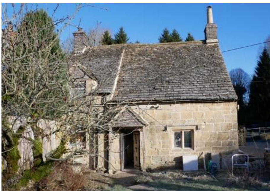
Plate 5: South elevation, C17 section to right with mullioned window fitted with a C19 metal casement
