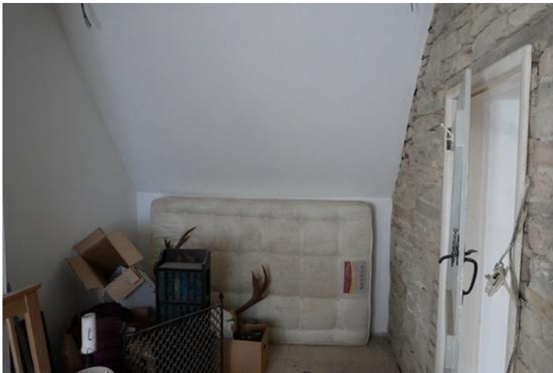
Plate 20: C19 section first floor room looking north
