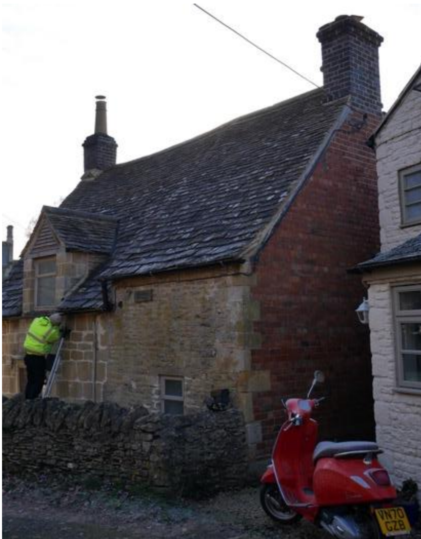
Plate 7: North and west elevations elevation, C19 section to right with higher eaves, coursed rubble and red brick walling and later C20
