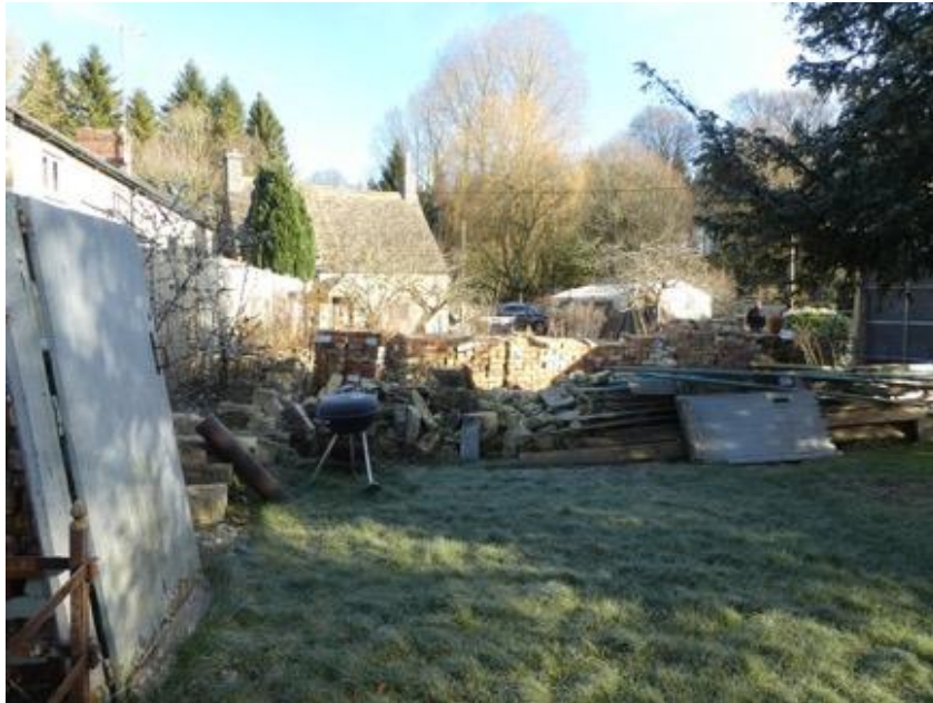
Plate 1: Garden to rear of Brookford Cottage with timber fence boundary to Brookside Cottages left, garden shed far right, garage beyond and Brookford Cottage centre
