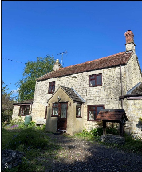
Plate 3. View of the cottage from the south
