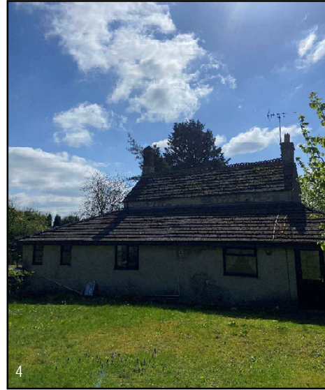
Plate 4. View of the cottage from the north showing single storey extension.
