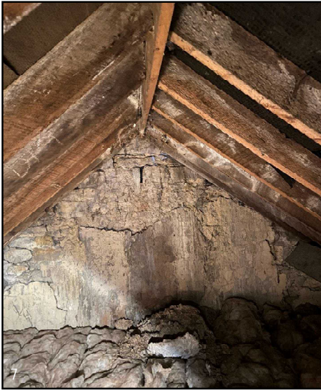
Plate 7. Internal view of the loft void in the Main Building
