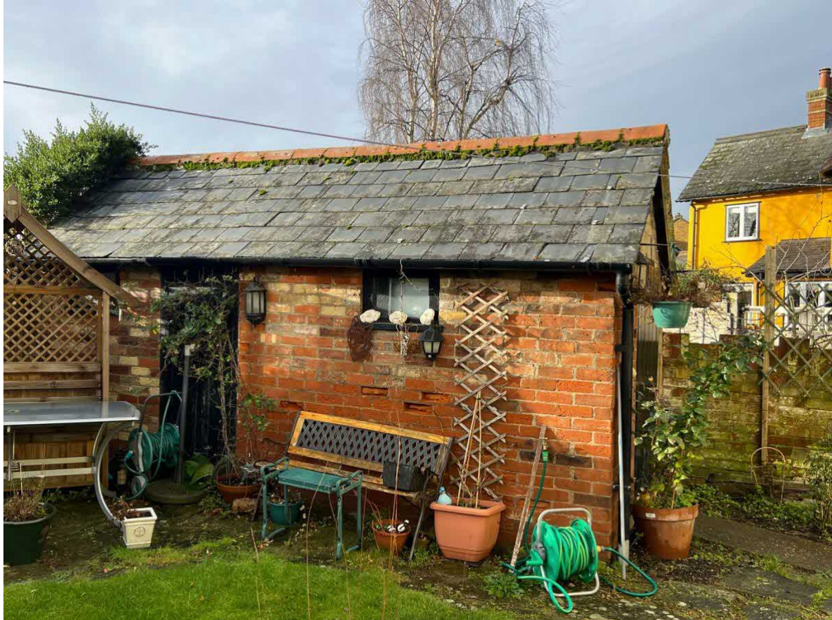
View of the outbuilding on site
