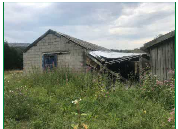
The southwest elevation of the lean-to and the outbuilding
