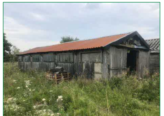
The southwest and northwest elevation of the outbuilding
