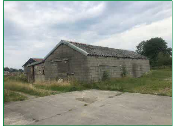
The southeast and southwest elevation of the barn
