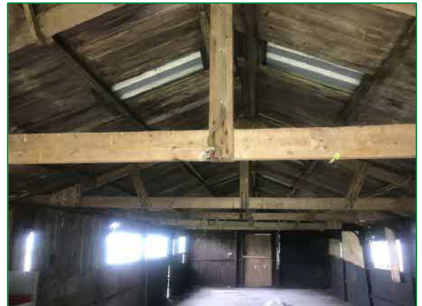
The interior of the outbuilding
