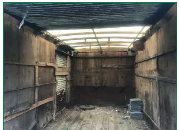
The interior of the shipping container
