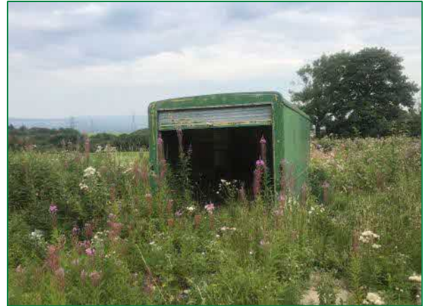
The southwest elevation of the shipping container
