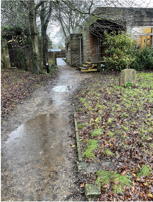
02 The resurfacing aims to reduce ponding by providing a permeable surface with a slight camber to direct surface water to the adjacent grass
