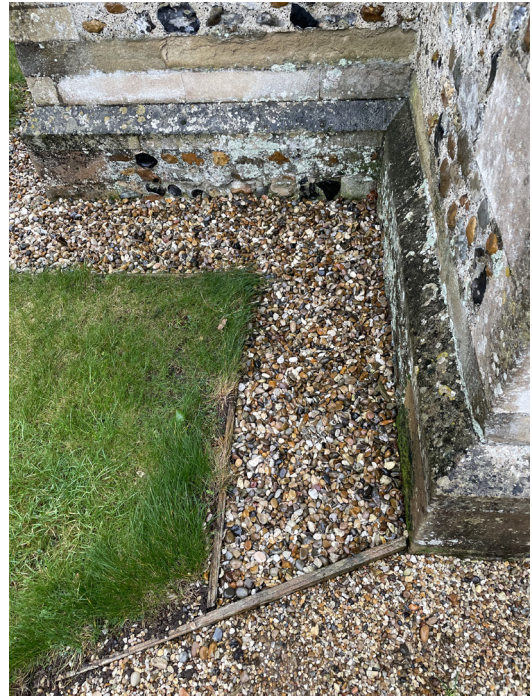
06 A free-draining gravel margin will be formed at the perimeter of the building in a similar way as the current arrangement at the west end.
