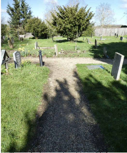
03 The paths have reduced in width because they have very few defined edges. The resurfaced paths will re-use existing masonry edging sections where these exist and treated softwood (sw) gravel boards elsewhere
