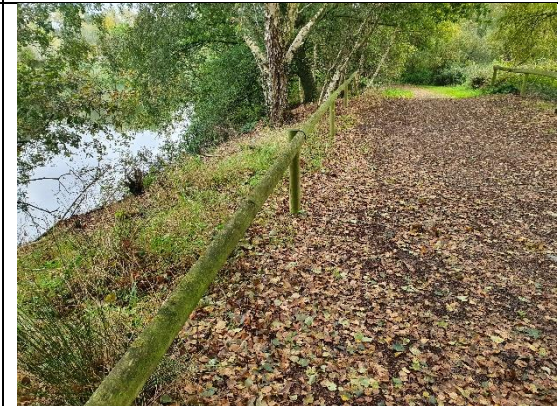
Photograph 3: Existing footpath on south side
