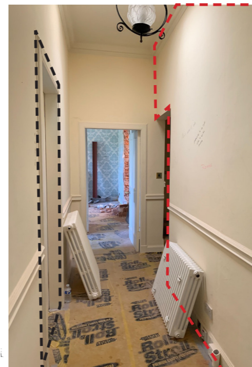
Original corridor. North-side wall removed and door on south wall blocked.
