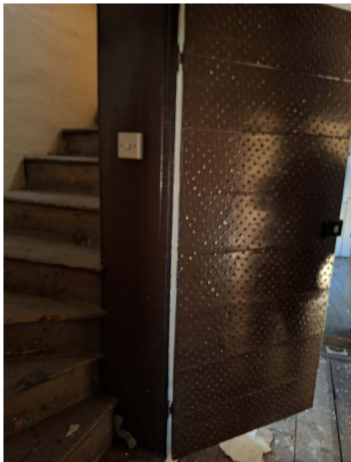
Stair to second floor
