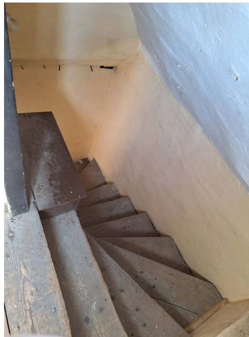
View of stair from second floor landing
