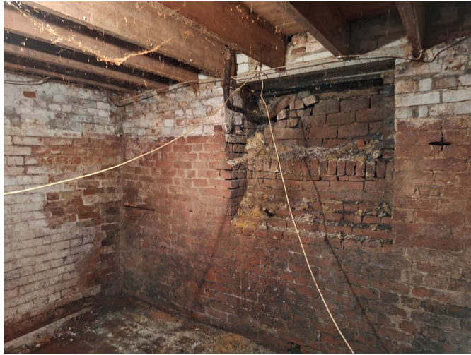
Existing basement bricked over lightwell
