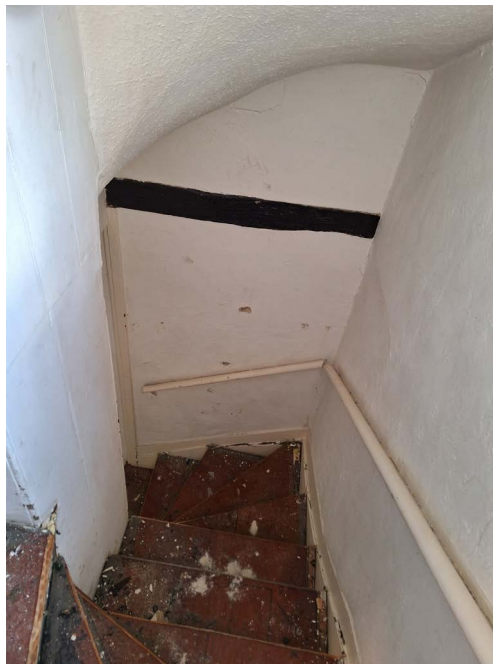
Stair to first floor
