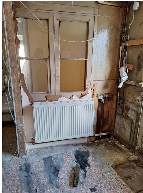
Existing c20 internal windows and partition wall to kitchen
