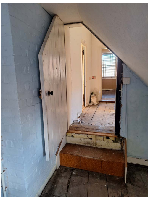
Existing Room 8 steps and view towards first floor landing
