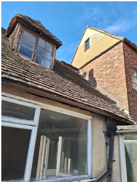
View towards dormer window to existing Room 8
