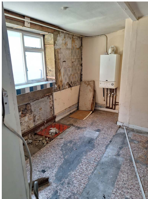
View of existing kitchen
