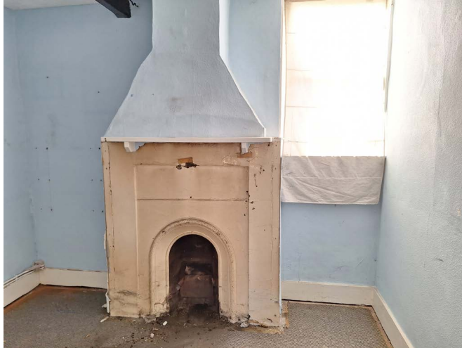
Existing Room 3 fireplace
