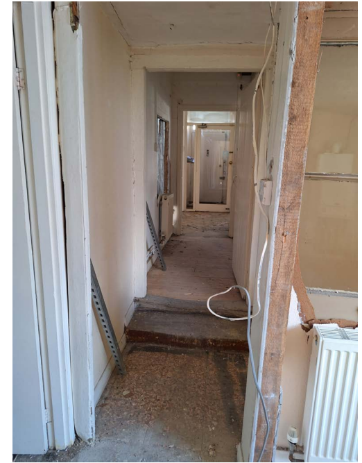
View along corridor from kitchen to front entrance lobby
