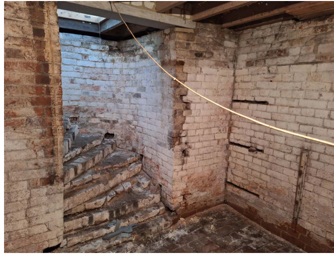
View back towards spiral brick stair to basement
