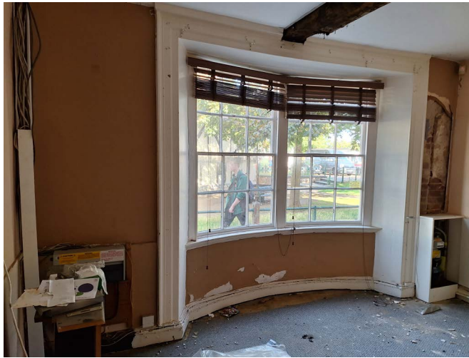
Existing Room 1 bay window to front
