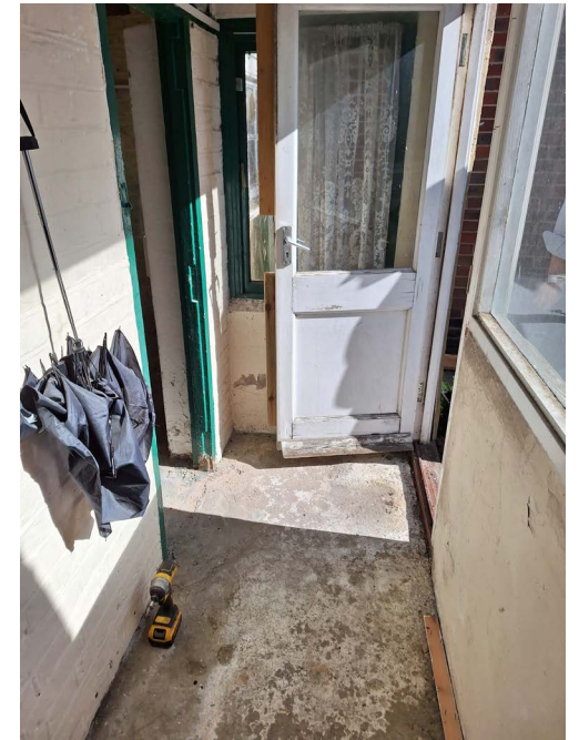
Rear lobby to existing single-storey rear extension
