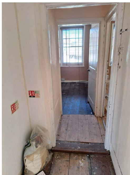
View towards existing Room 6 from the first floor landing
