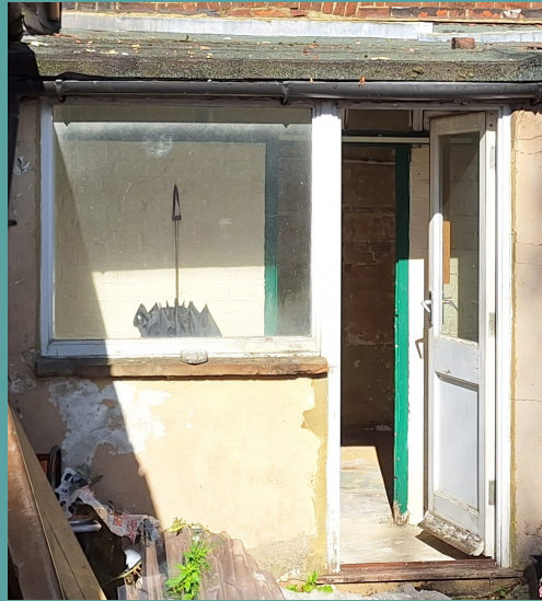
7 Existing window serving ground floor lobby
