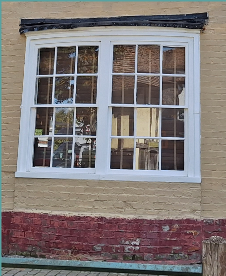
1 Existing window serving Room 1
