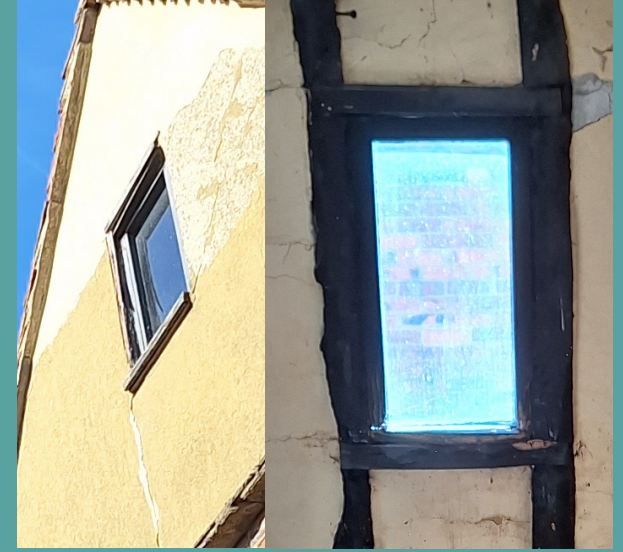
19 Existing window serving second floor landing
