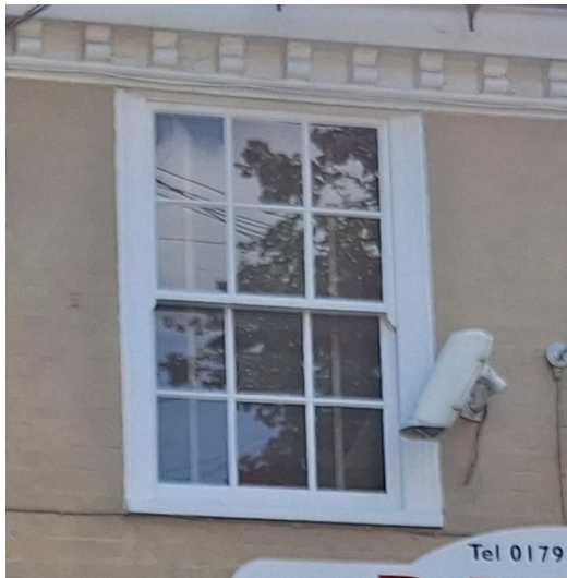
12 Existing window serving Room 6
