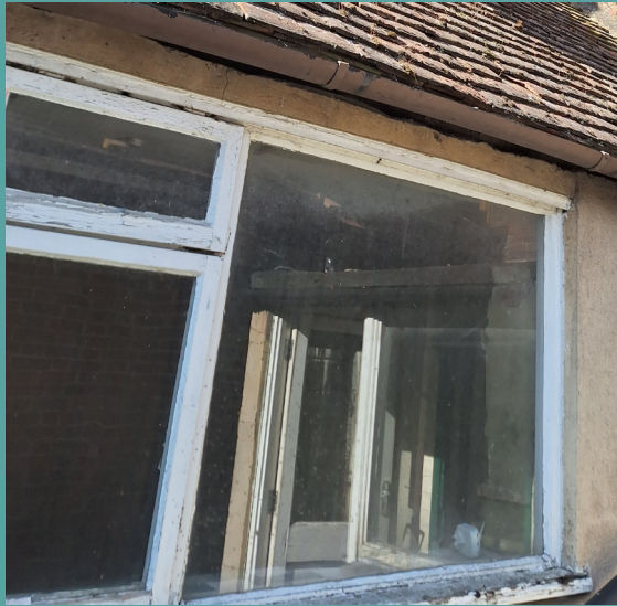
Existing window serving Kitchen (partial external view)
