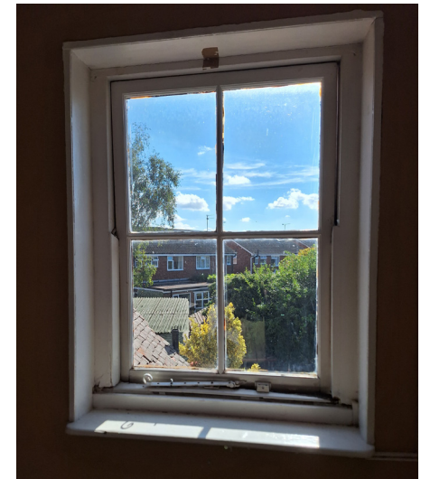
14 Existing window serving Room 7
