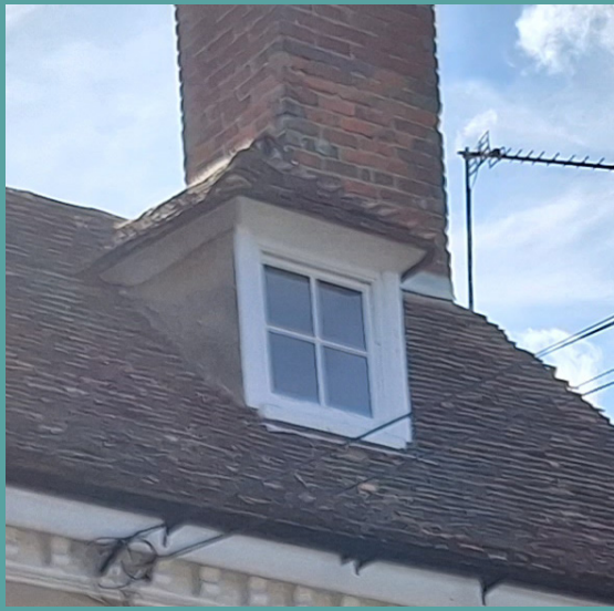
18 Existing window serving Room 10
