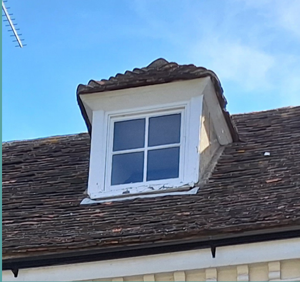
17 Existing window serving Room 9
