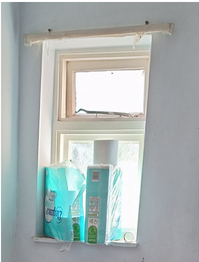
4 Existing window serving WC
