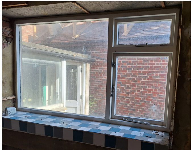
6 Existing window serving Kitchen
