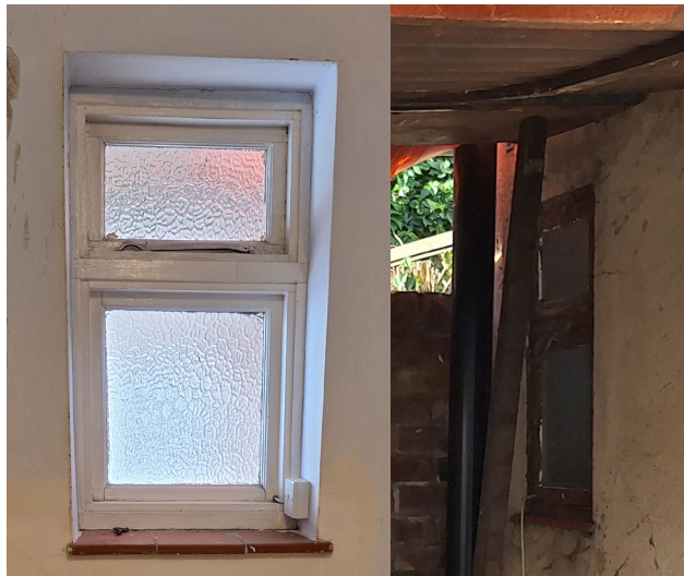
5 Existing window serving Staff Room
