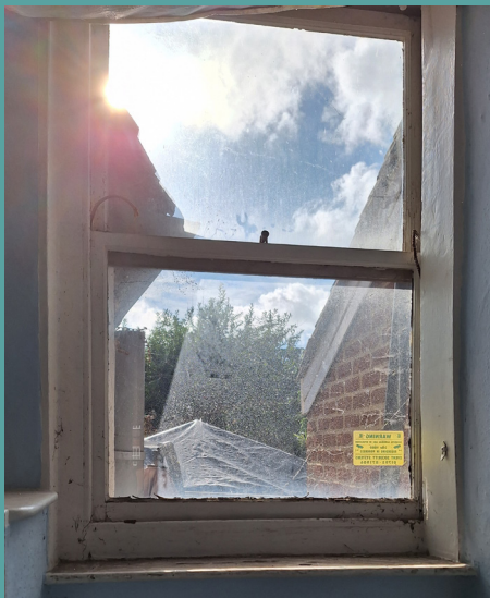
3 Existing window serving Room 3
