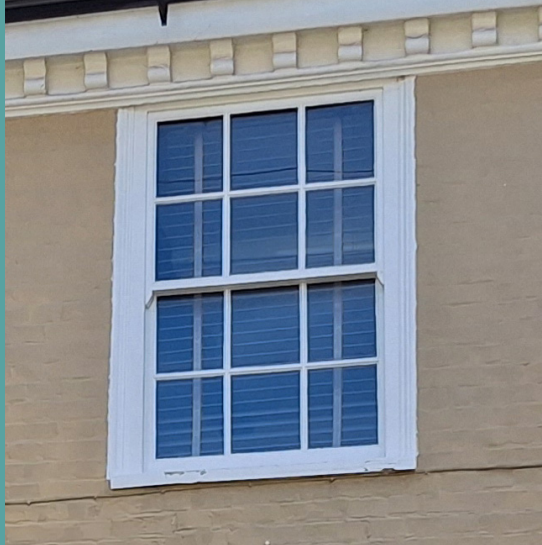
10 Existing window serving Room 5
