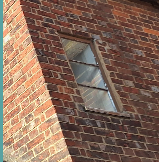
16 Existing window serving stairs
