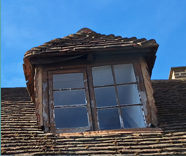
15 Existing window serving Room 8
