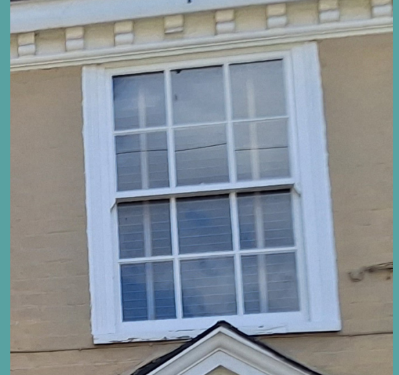
11 Existing window serving Room 6
