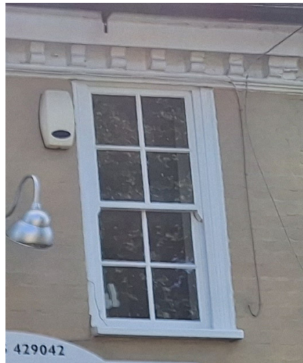
13 Existing window serving Room 6 (cupboard)
