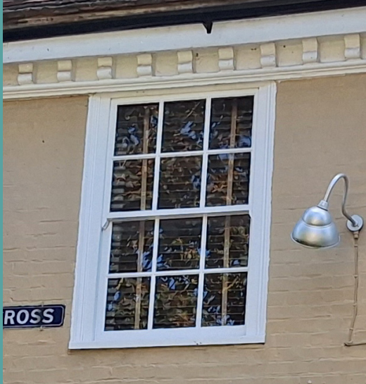
9 Existing window serving Room 5
