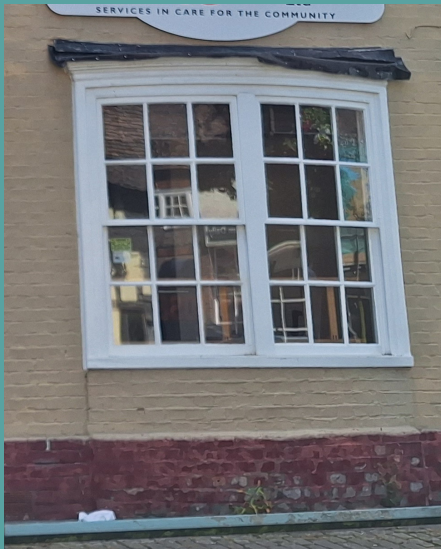
2 Existing window serving Room 2
