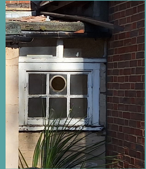
8 Existing window serving Room 4
