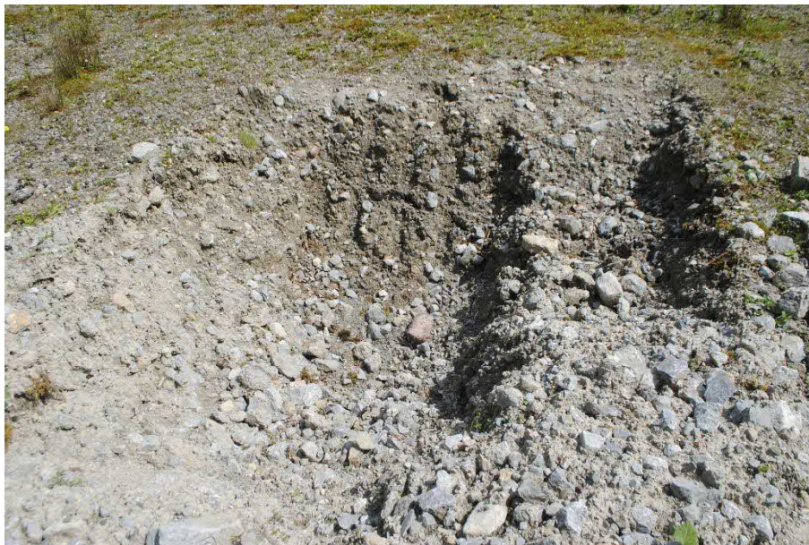
Figure 6.1. Showing existing hardcore base
