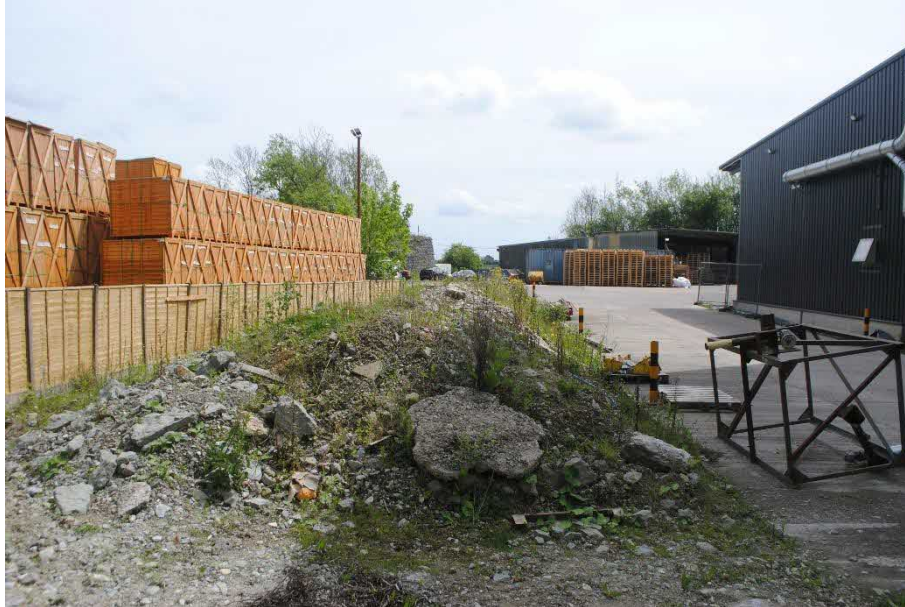
Figure 4.8. Bund to be removed.
