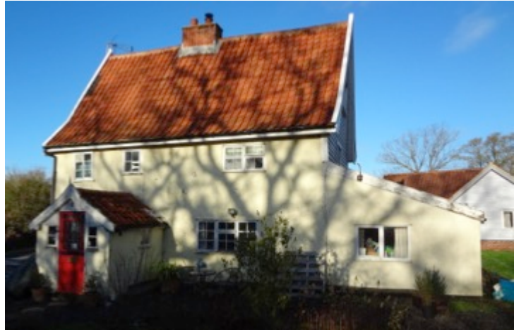
Photo Front South (view from drive) Elevation
