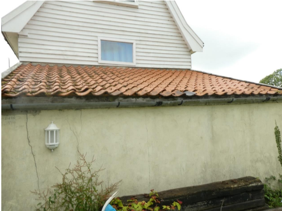
Photo 3 , looking northwest towards the eastern extension.
