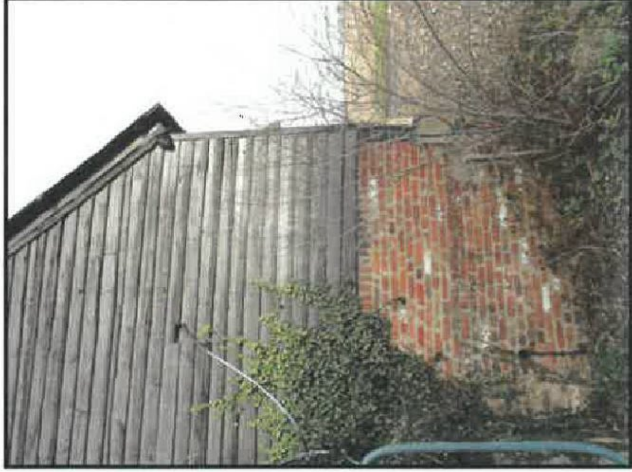
South-West Side Elevation - Photo 14
