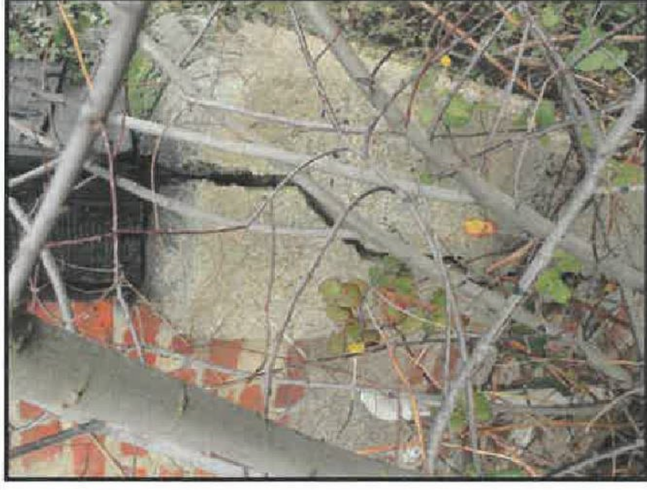
South-West Side Elevation - Photo 15
