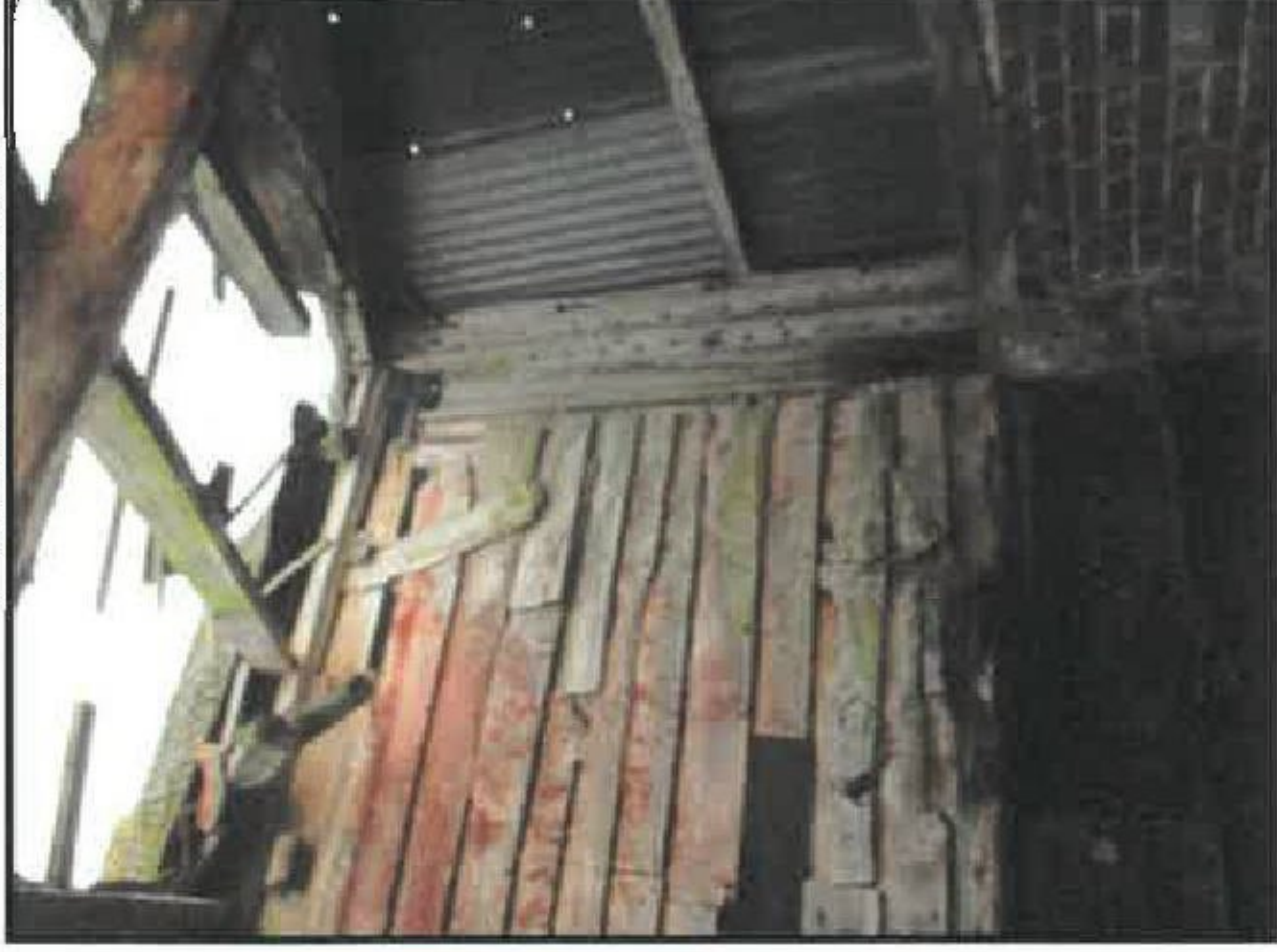
North-West Side Elevation - Photo 26
