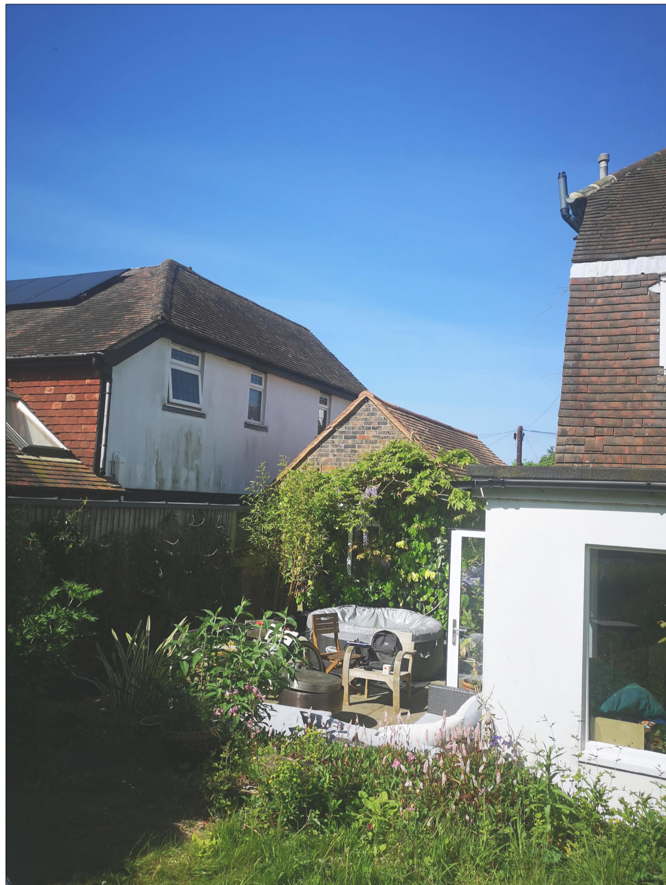
Photo 3 - Rear of garage - no.2a Surrenden Close to left
