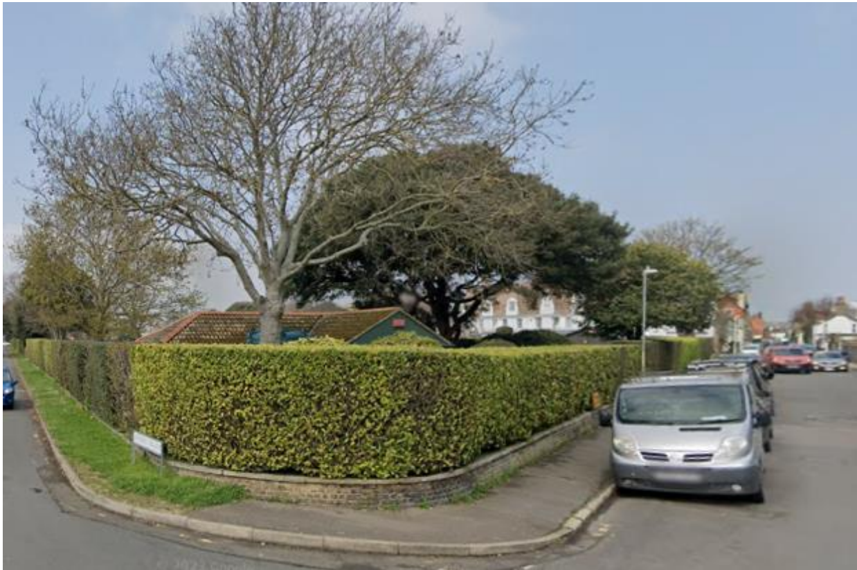
Figure 20: Single-storey structure in southeastern corner of Archery Gardens
