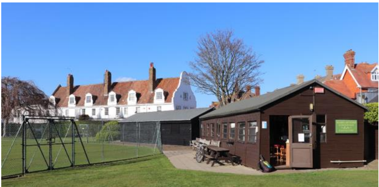
Figure 19: Existing structures at east end of Archery Gardens
