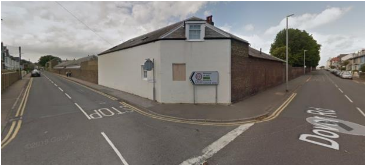
Figure 17: Building 129 Guard House
