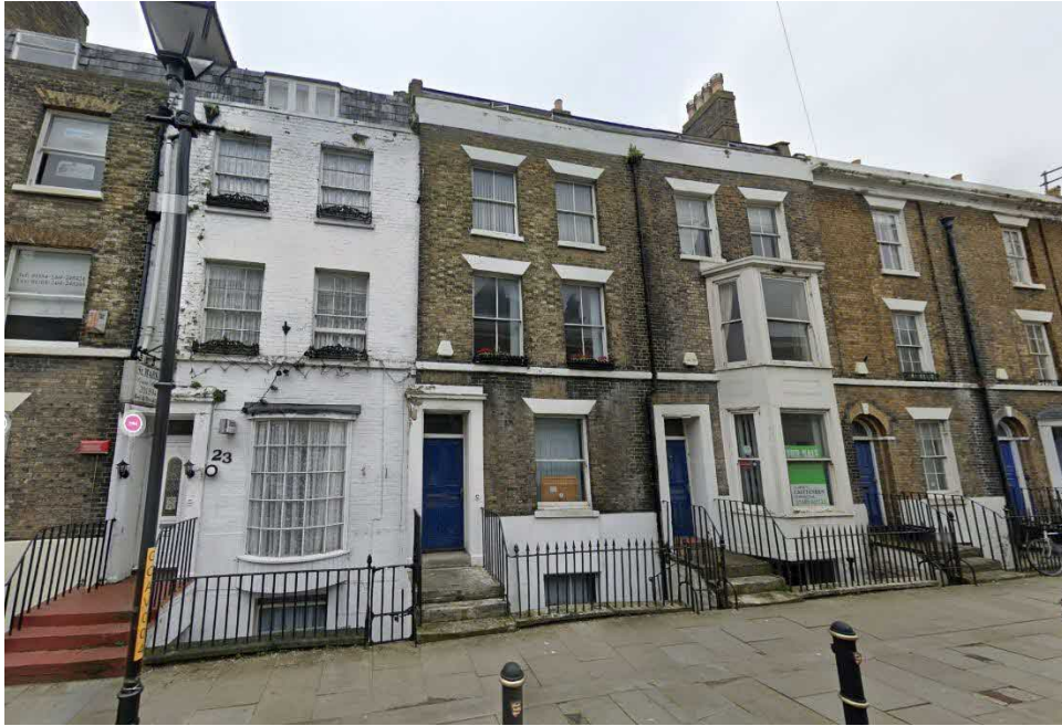
Fig 1. Street elevation. No.21 is in the centre property.
