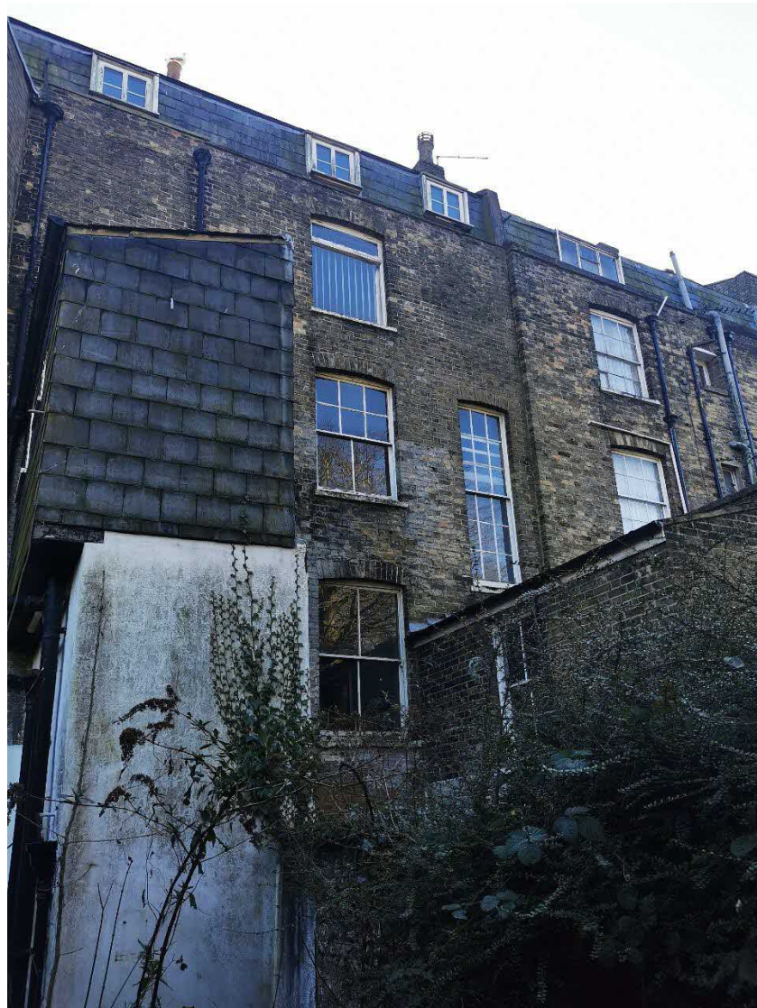
Fig 2. Rear elevation. No.21 is the centre property.
