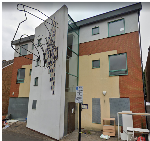
Figure 1 - Front Elevation of 162 Gillet Road
