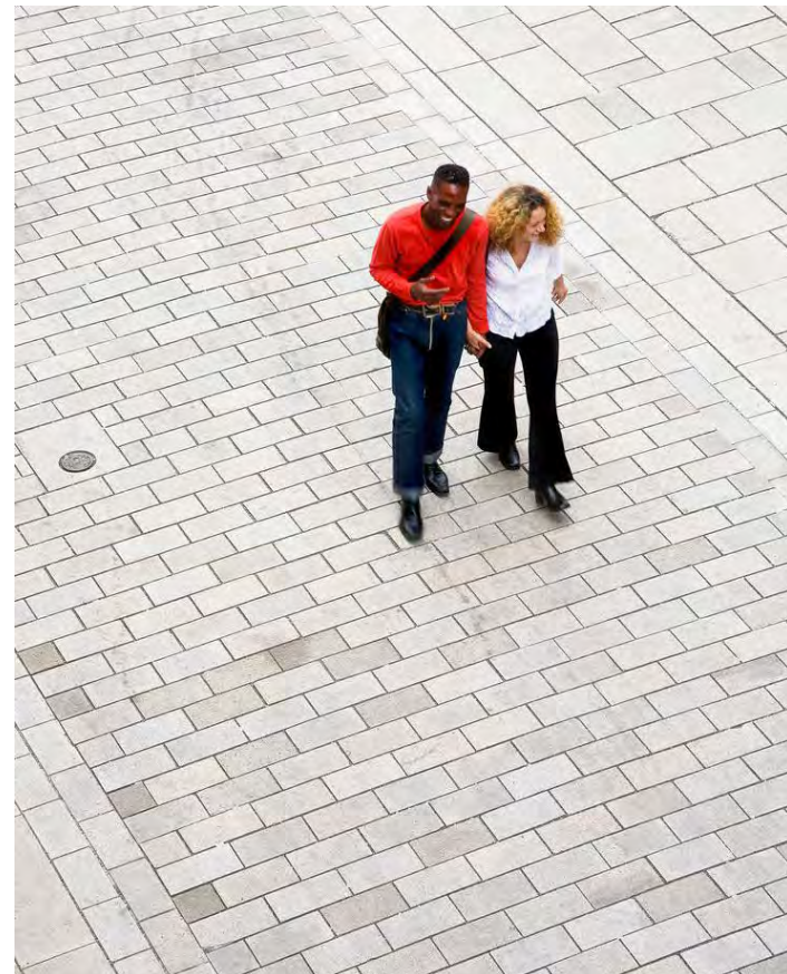
Shared surface in natural stone block paving
