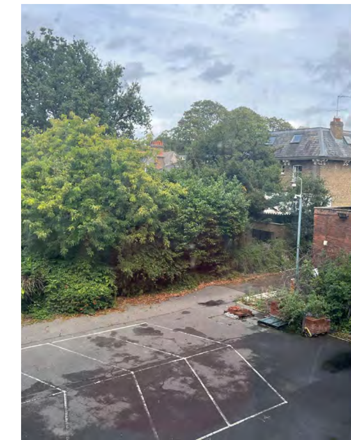
Existing asphalt in the Copper Beech Courtyard
