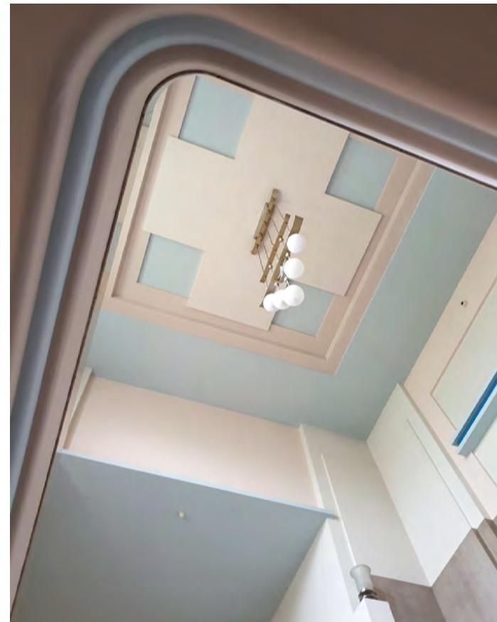
Existing ceiling in Block A
