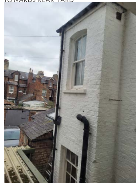
VIEW FROM UPPER FLOOR WINDOW LOOKING TOWARDS REAR PROJECTION
