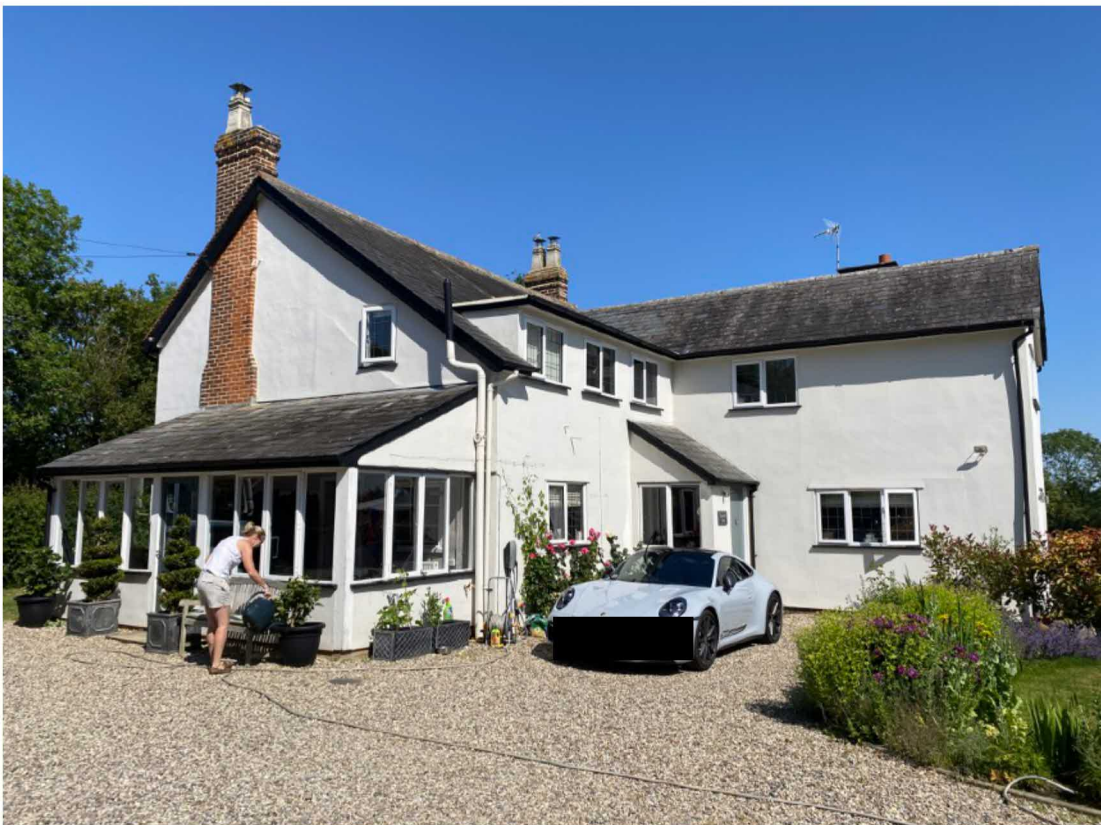
Side View (Looking North)
