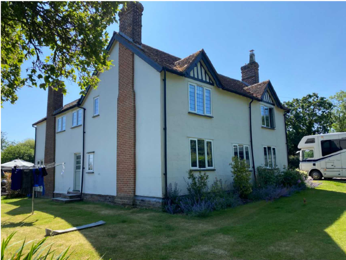
Front View (Looking South East)
