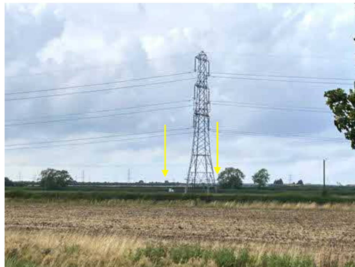
4. VIEWPOINT 1: GREAT NORTH ROAD (EAST): Zoom of Photo 3. The location of the application site is highlighted between the two arrows.
