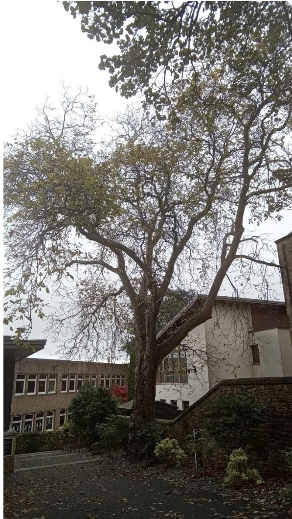
WALNUT (2224) IN CLOSE PROXIMITY TO SURROUNDING BUILDINGS WITH RECENT BUILDING WORK IN ROOT ZONE AND POSSIBLE HOLLOWING OF MAIN STEM
