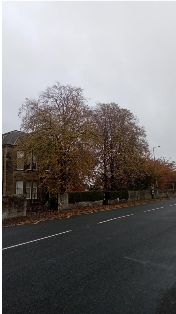
4 X LIME (2222) EXHIBITING HISTORIC TOPPING WOUNDS NOT FULLY VISIBLE FROM GROUND LEVEL
