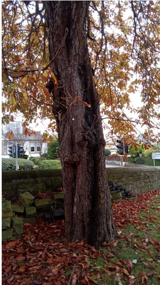
CHESTNUT (2220) EXHIBITING BURIED BASAL FLARE ABOVE RETAINING WALL WITH POSSIBLE STEM HOLLOWING
