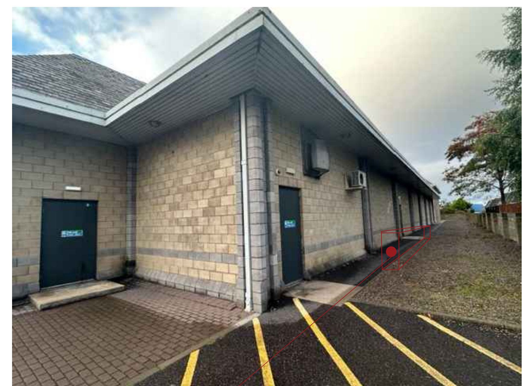
EXTERNAL Power Inverter Heat Pump PUZ-ZM200-250 R32 6 No Mounted on shoes at ground level.
