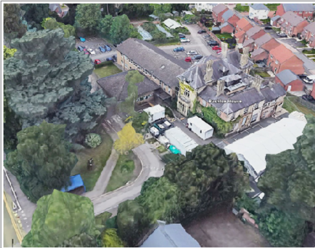
Figure 2: Bushloe House and its associated outbuildings
