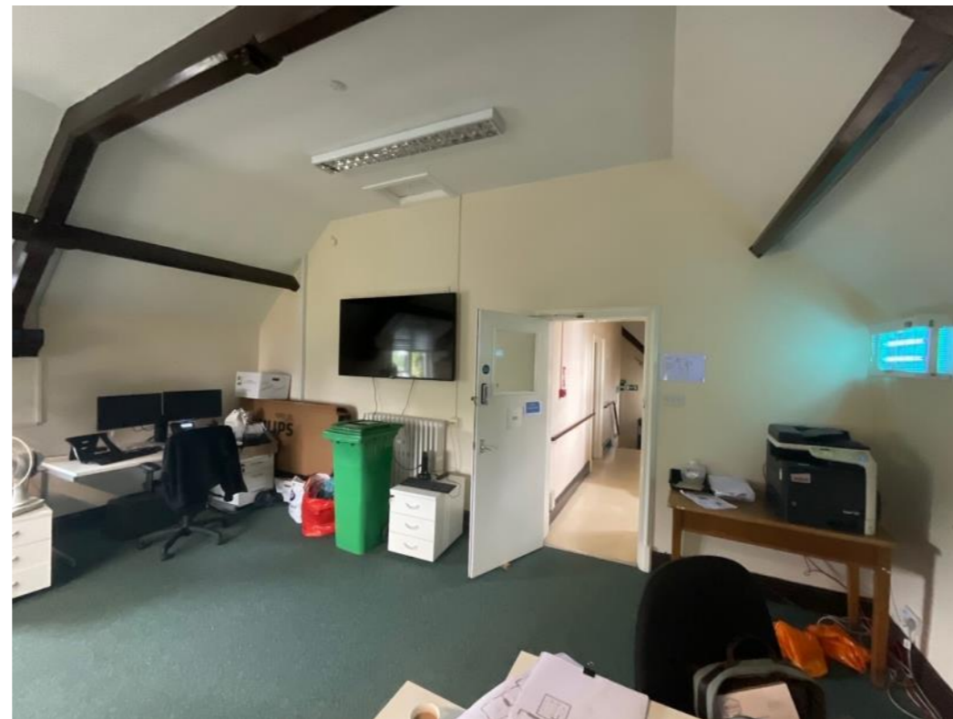
Figure 23: Suspended ceiling to second floor
