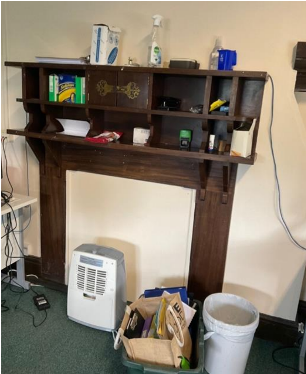
Figure 18: Wooden fireplace with smokers box
