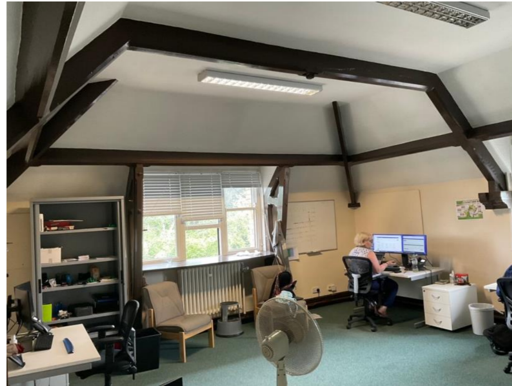
Figure 22: Suspended ceiling to second floor
