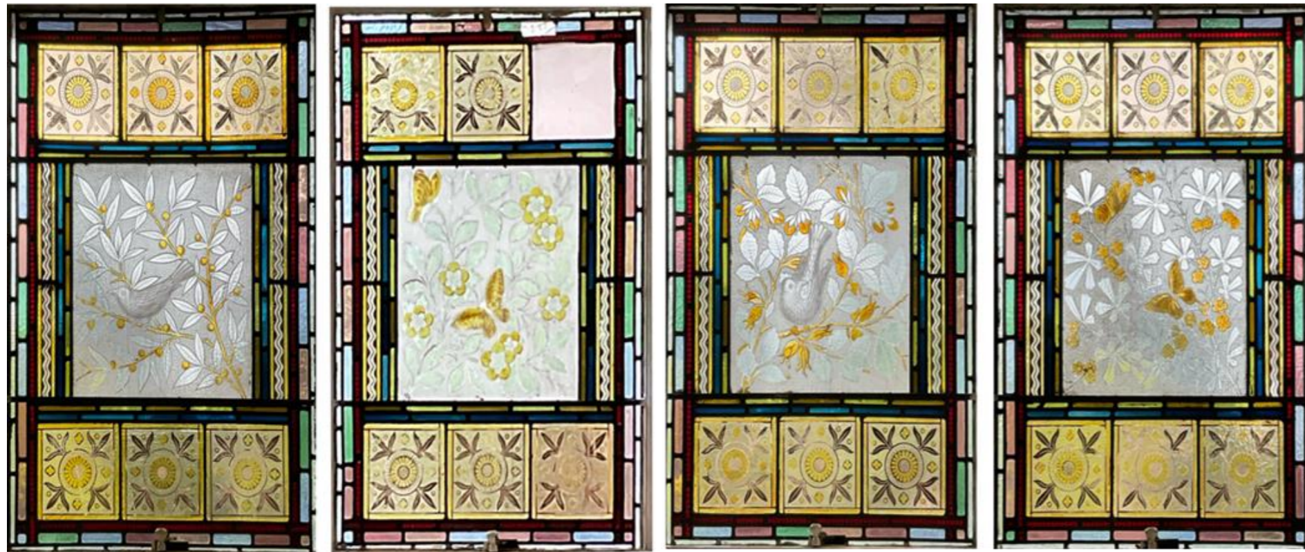
Figure 9: Stained glass - oriel window centre panels (x4)
