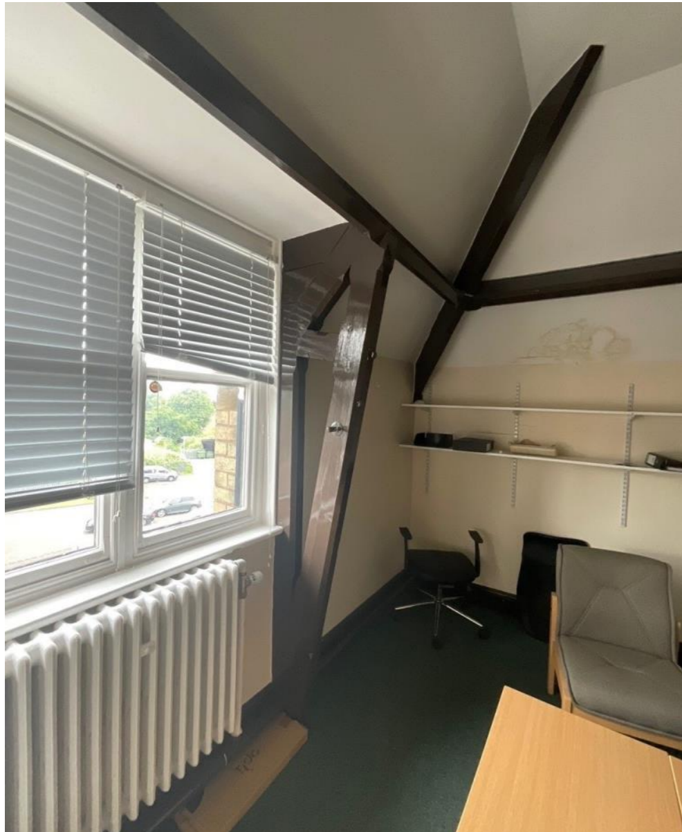
Figure 21: Suspended ceiling to second floor
