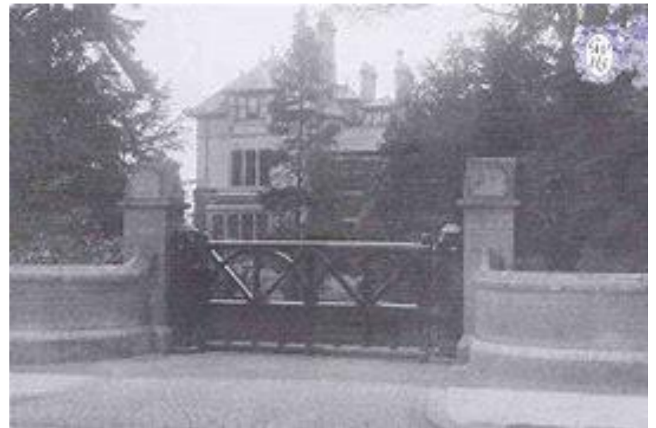
Entrance gate and posts with perimeter wall once in place.
