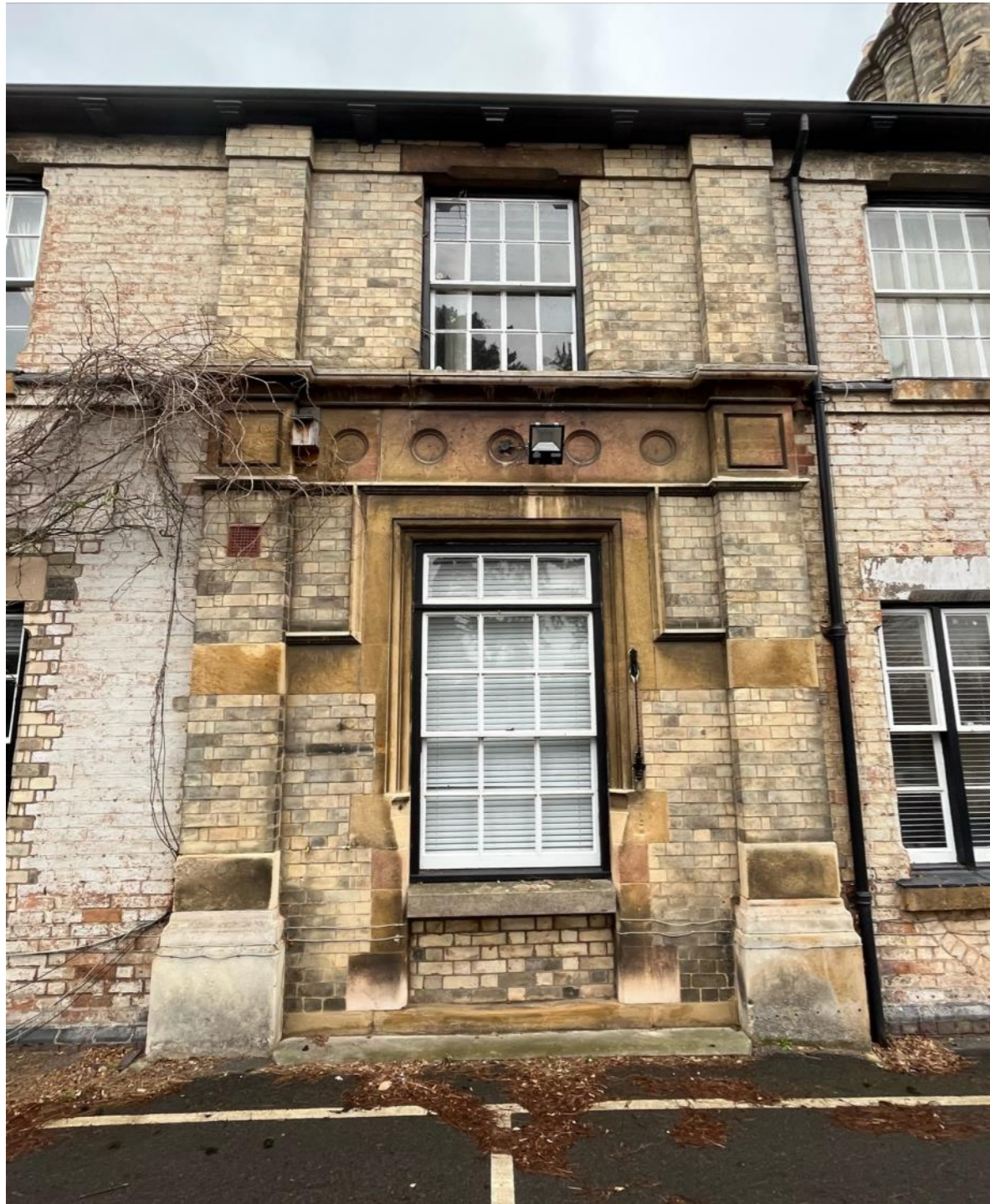
Figure 13: Original front door, now filled
