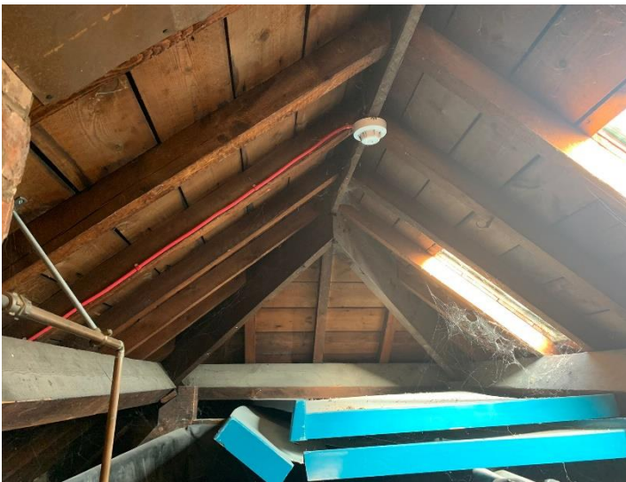
Figure 3. An Internal loft void within the main building
