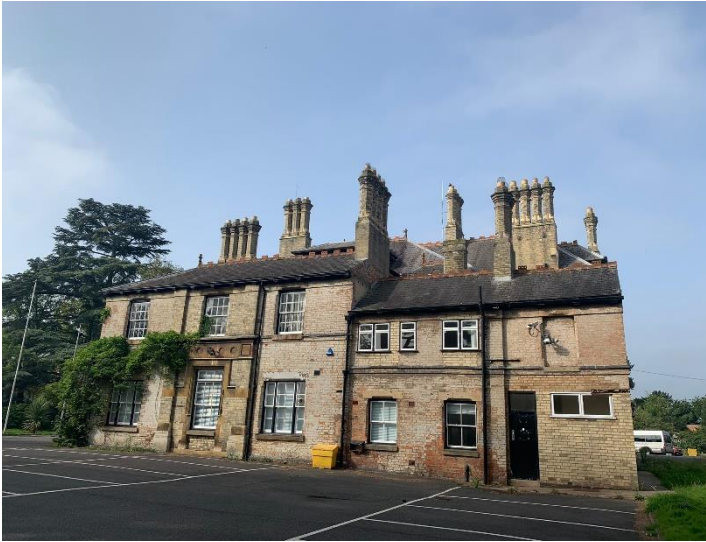
Figure 1. Eastern elevation of the main building
