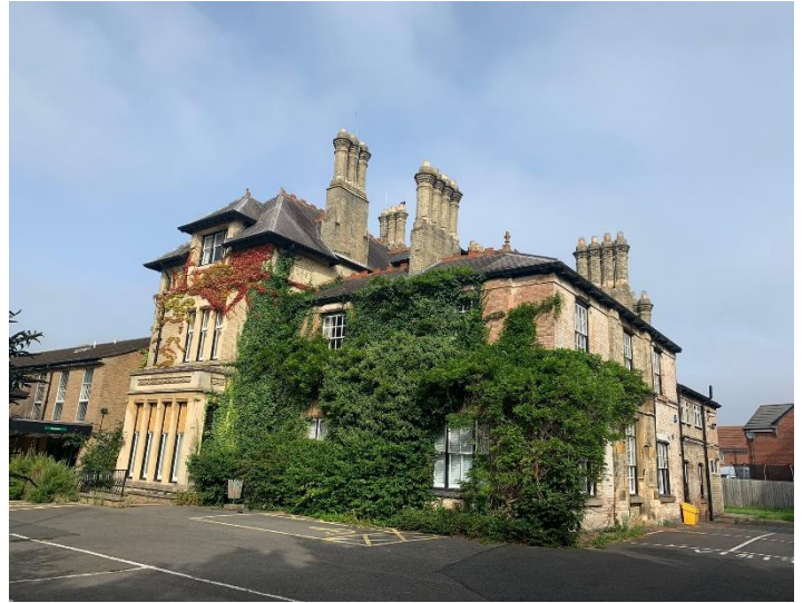
Figure 2. Southern elevation of the main building
