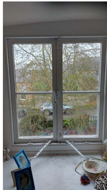
Internal of existing timber window
