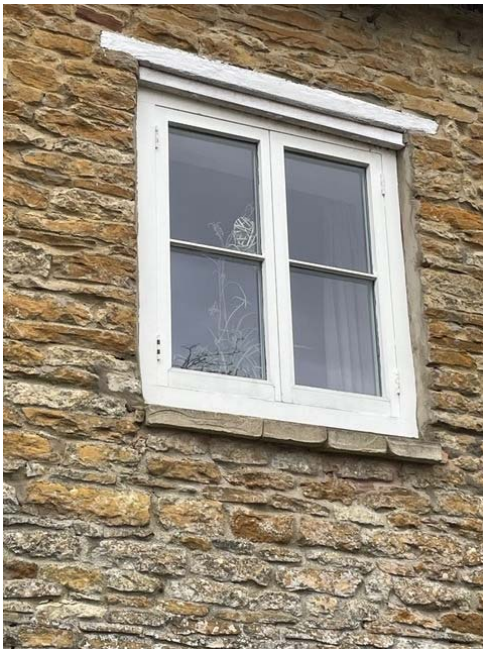
External of existing timber window
