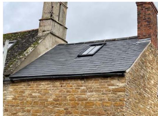
To match one already installed on existing
