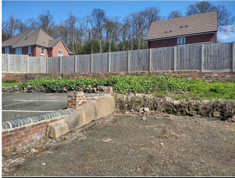
View towards recently completed adjacent Housing development (Picture 3)
