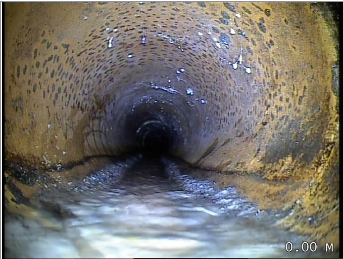
Start node type, manhole, reference MH1
