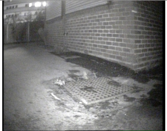
Manhole / Access Point: MH1 Location
