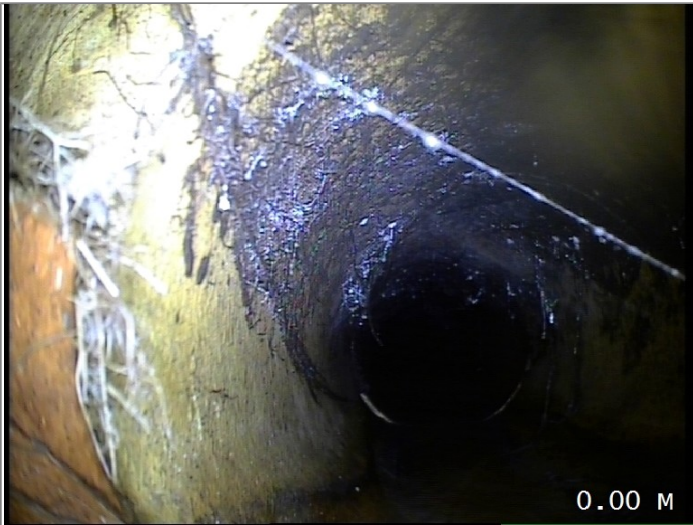
Start node type, manhole, reference MH2 BURIED
