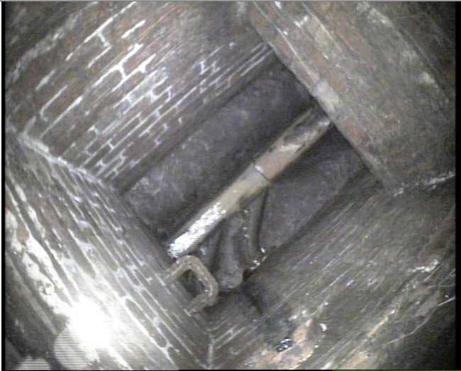
Manhole / Access Point: MH1 Internal
