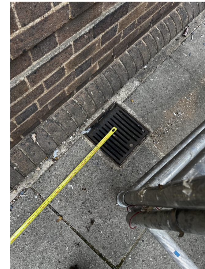
Image of Existing Brick Vents and Gratings Scale: 1:20 at A1
