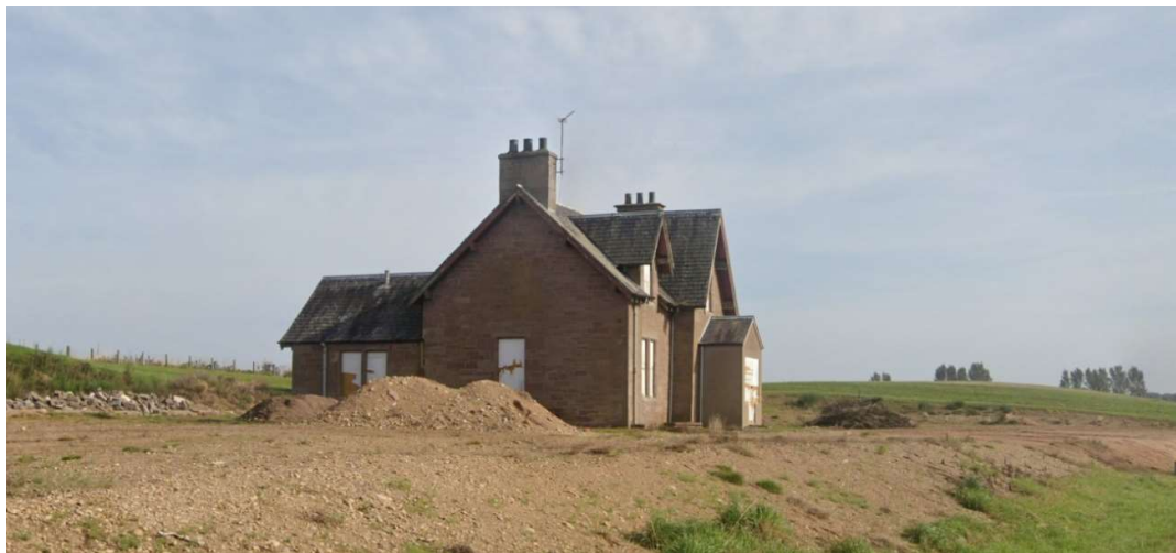
Side elevation following demolition works on adjacent plots
