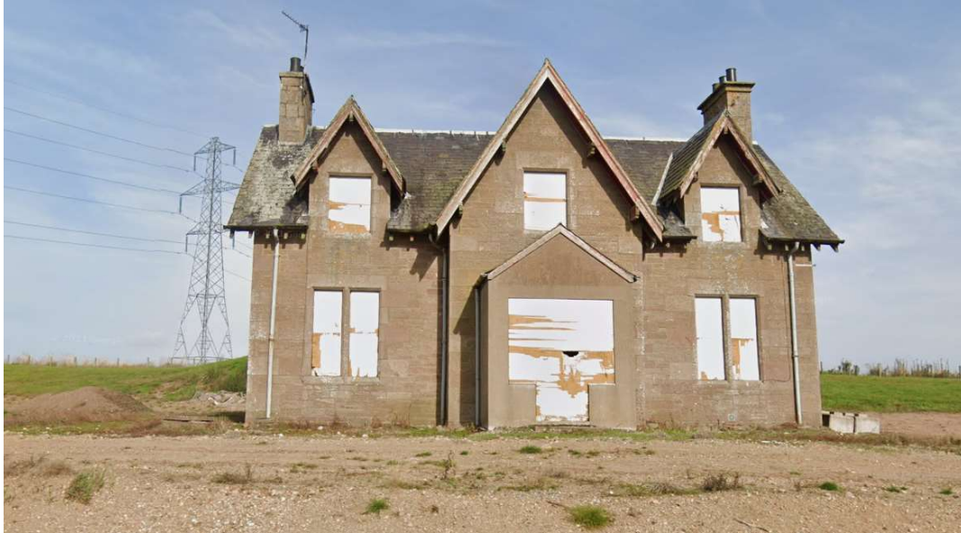
Front elevation following demolition works on adjacent plots
