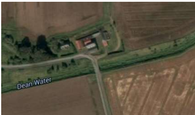
Site prior to the demolition of the steading and storage units.
